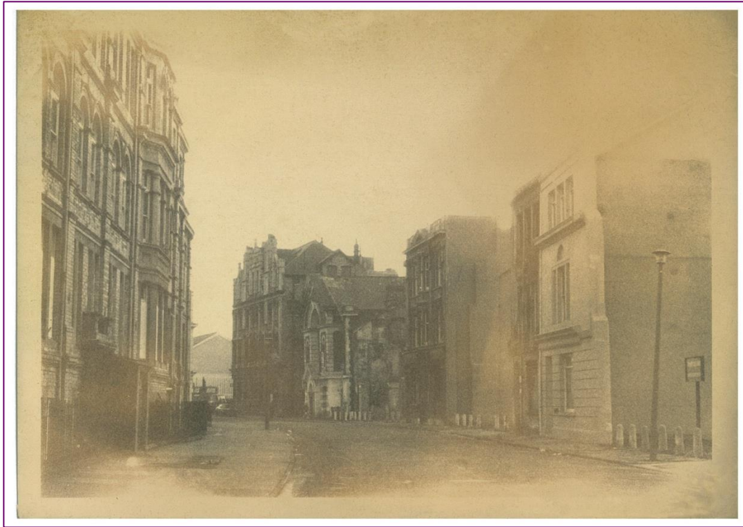
The Casablanca Club in Mount Stuart Square, Cardiff Docks, circa 1970. The club is the old chapel building (centre). I took this photo for the Cardiff student newspaper Broadsheet, of which I was editor. The Casablanca was demolished in the 1990s.
