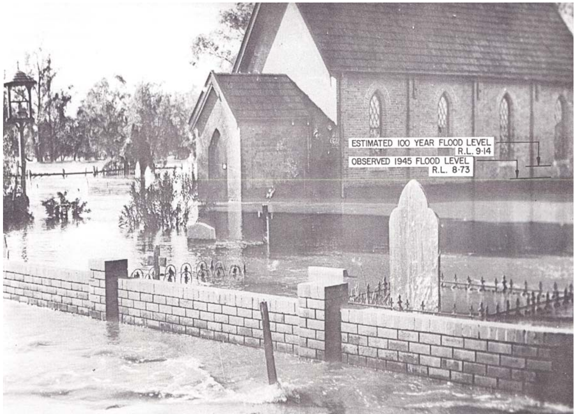
Figure 3-6: Flooding Around St John's Church, Pinjarra – June 1945 (Richards, cited in George 1984)
