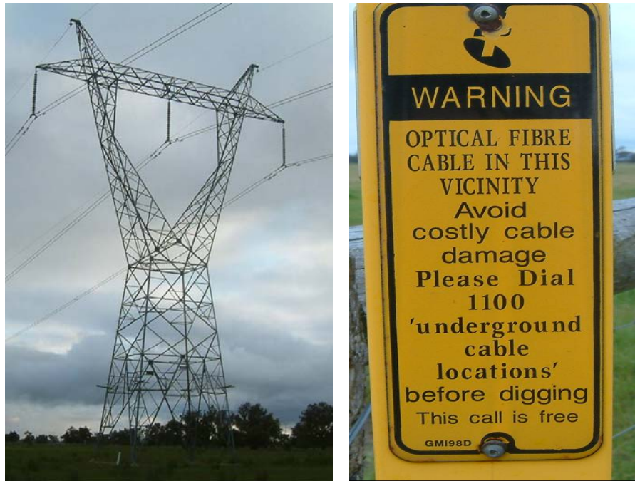
Figure3-18: Existing Services at the Proposed Diversion Channel
