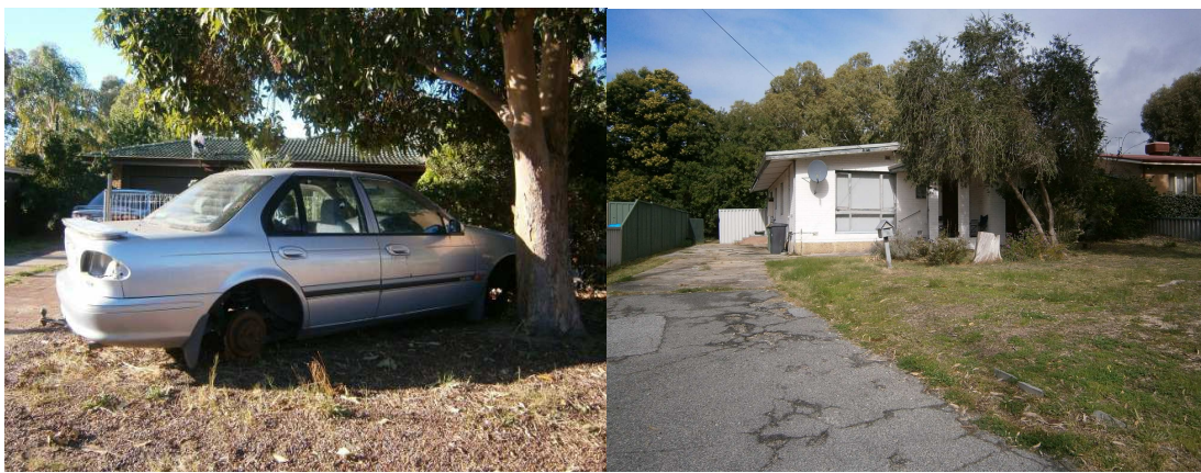
Figure 104 and 105: Many existing dwellings in the study area were observed in poor condition, reflecting a low maintenance standard, both pre- and post-redevelopment (Author 2014).
