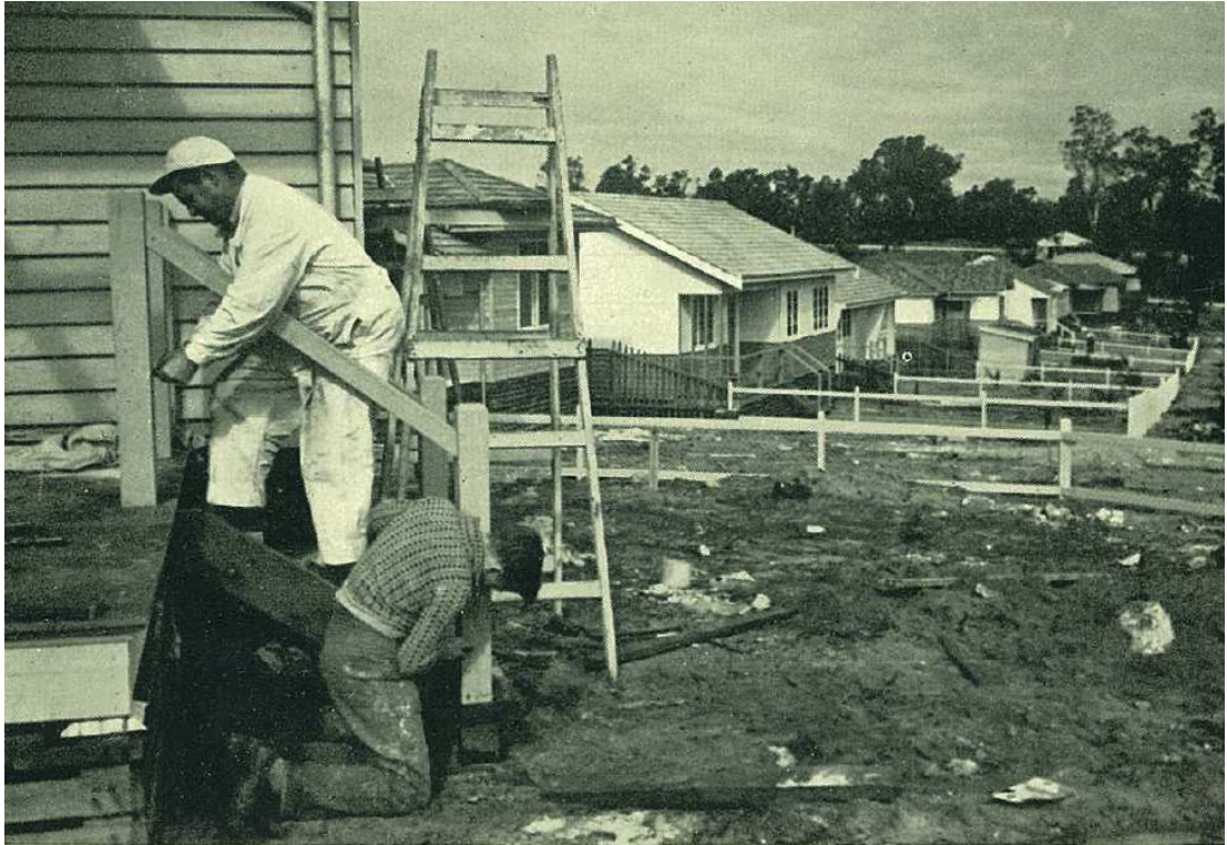
Figure 30: Workmen engaged on the State Housing Commission project at Medina on the periphery, the first neighbourhood of the Kwinana New Town (Stephenson and Hepburn 1955, 24).
