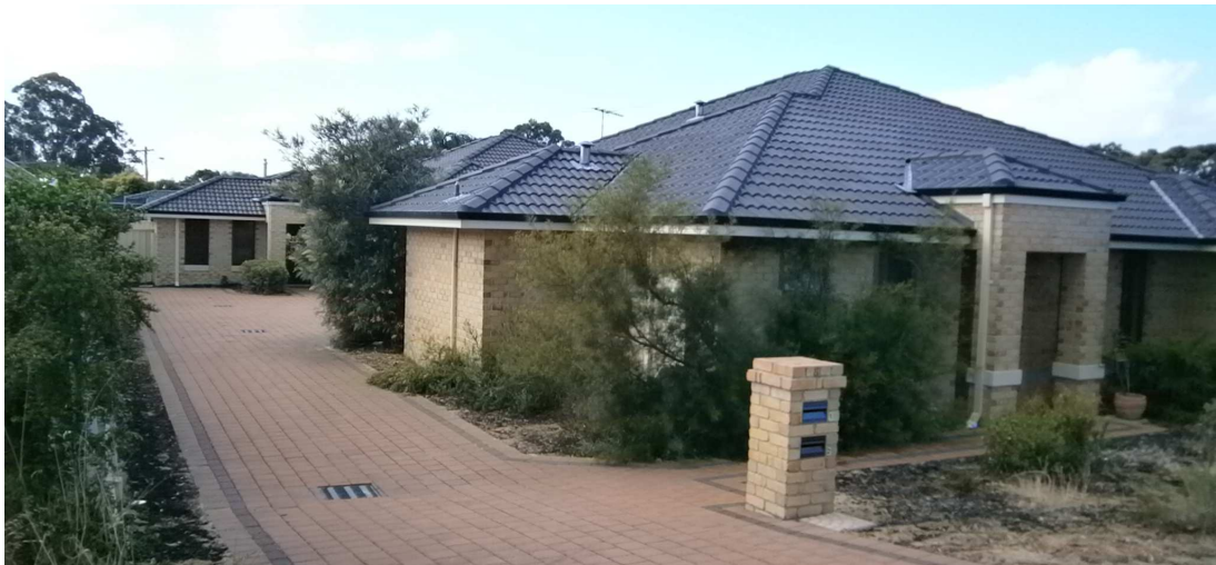
Figure 111: New dwellings along prominent Third Avenue (Author 2014).
