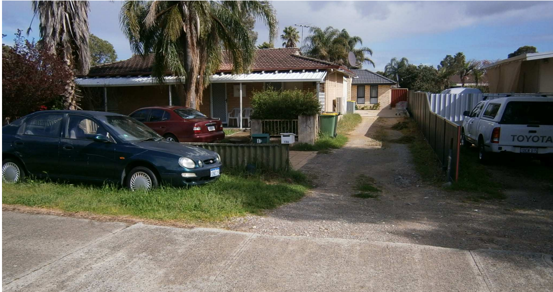
Figure 122: Poorly executed battleaxe redevelopment, Merrifield Avenue Kelmscott, located approximately 500m from the Kelmscott Train Station (Author 2014).
