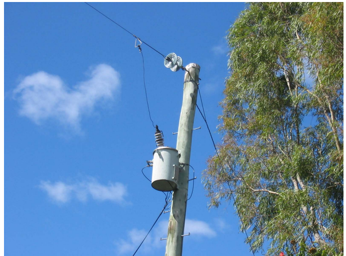
Fig 1. A Single Wire Earth Return Consumer Connection Transformer
