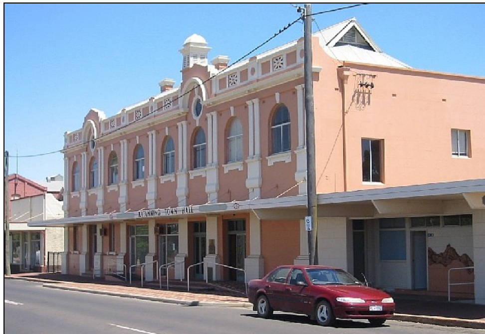
Plate 5: Katanning Town Hall, in the process of being renovated, will include office facilities for an Indigenous Community Arts Officer.
