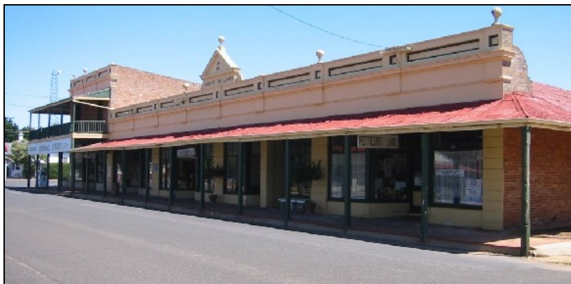
Plate 7: Jones Building currently being renovated to house a bakery and wine cellar, town of Broomehill
