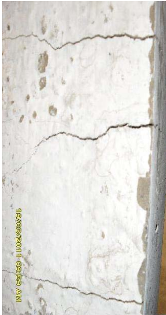
(a) Cracks on tension sides
