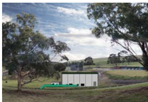
Figure 3.4 Greenvale Pumping Station (Water Corporation, 2011)
