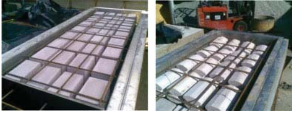
Figure 2. Construction of LSRC slabs.
