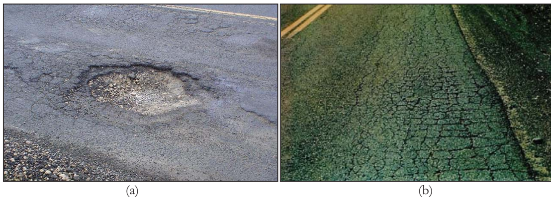
Fig. 2. Deteriorated pavements due to Water induced damage, (a) pothole (b) alligator cracking [2].
