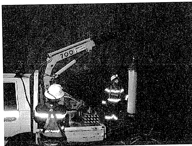
Fig. 1. VOIS and its deployment system mounted on LV
