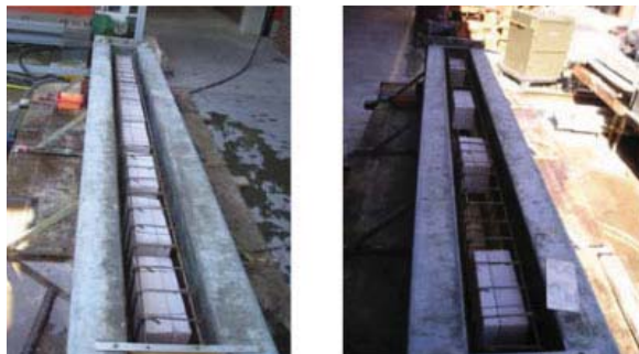
Figure 1. Construction of LSRC beams.
