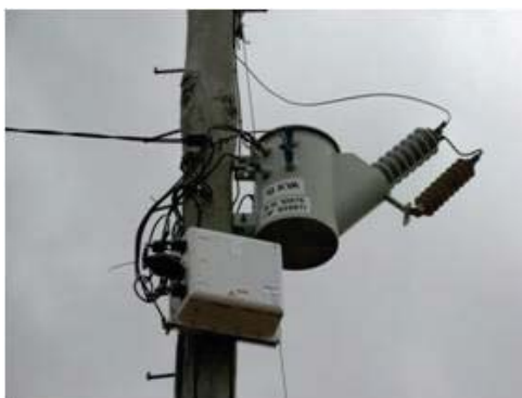
Fig. 1. LVR installed on a SWER [1]
