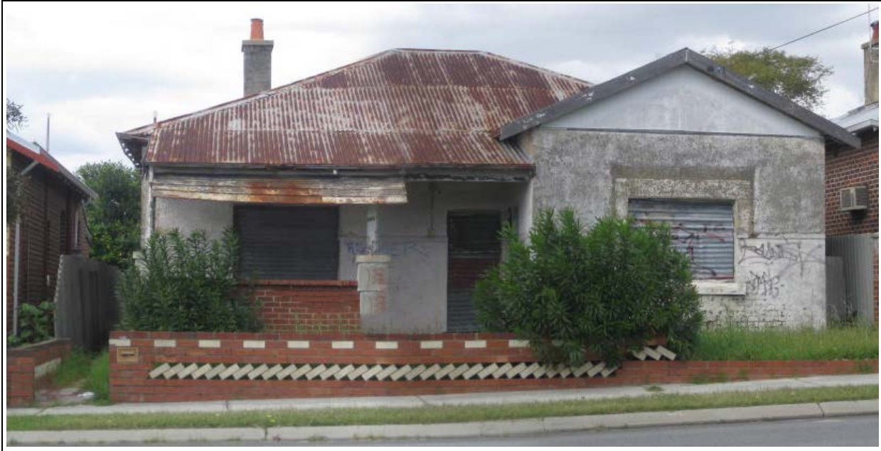
Figure 4. Vacant / poorly-maintained ‘House A’ (Anonymous, 2008)
