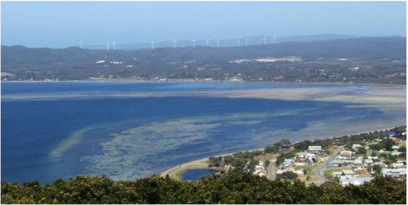
Photo of Albany Wind Farm from Albany city
