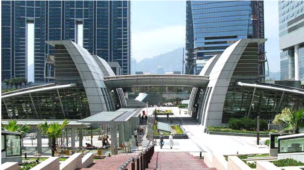
Figure 3.24 Kowloon Station, Hong Kong
