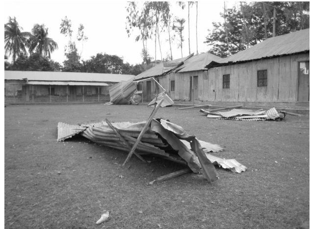
Fig. 3. Roofs of Dogasi school and college in Jamalpur blown off by wind gusts associated with a severe local storm on April 26, 2010, in Jamalpur, Bangladesh.
