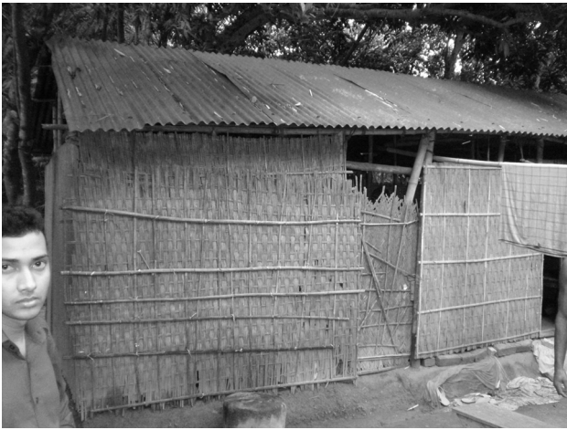
Fig. 2. The house of a local interviewee in our survey of the severe local storm event on September 5, 2008, in Jamalpur, Bangladesh.
