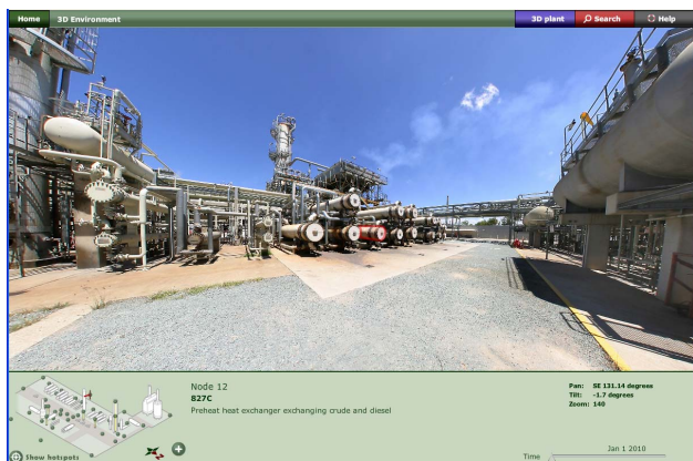
Figure 4. View of heat exchangers in the Virtual Process Plant
