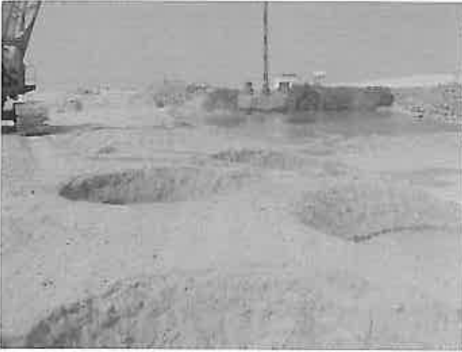
Fig. 9. Dynamic Compaction Craters.
