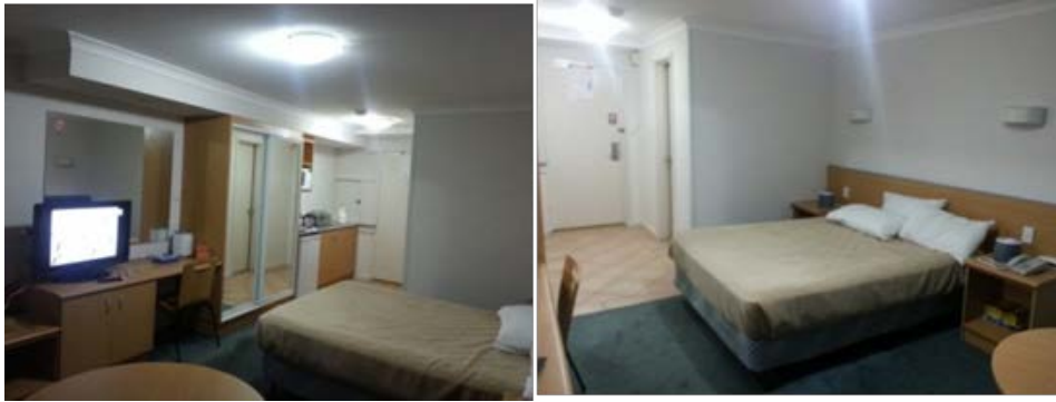
Figure 7.3 The general ceiling white lighting and the wall white lighting fixtures over the bedside tables.
