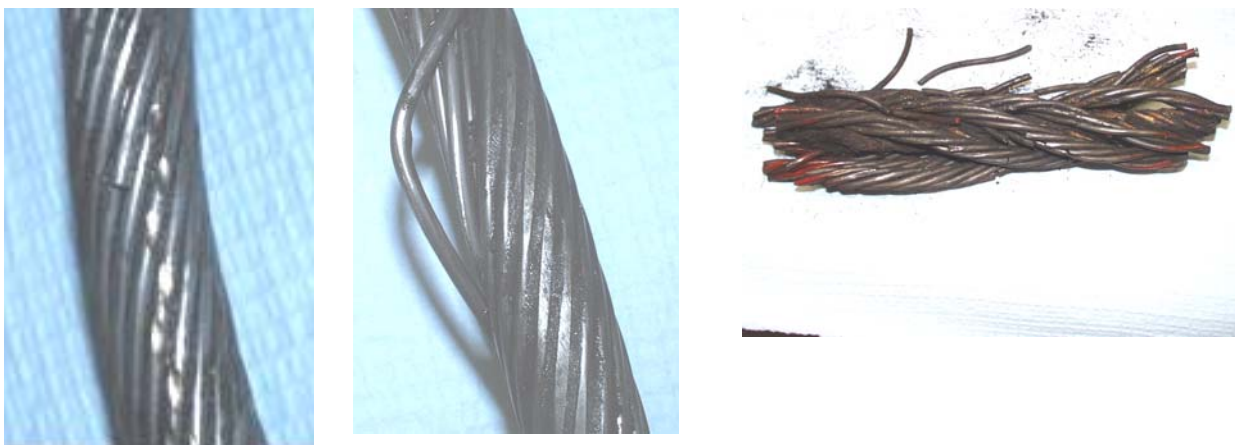
(a) Indented Wires – Inside of Strand (b) Worn out Wires – Outside of Strand (c) Core – Wires Broken into Small Pieces
