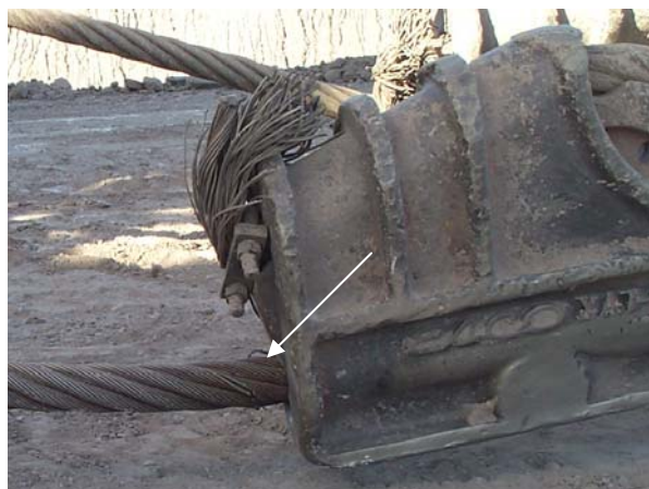
Figure 4: Typical Wire Breaks at Sockets
