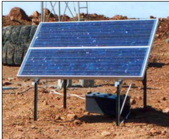
Figure 4.15 Solar panel array
