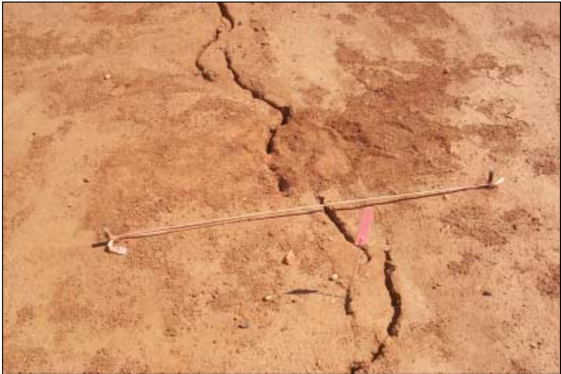
Figure 2.5 Pin crack meter measuring crack displacement
