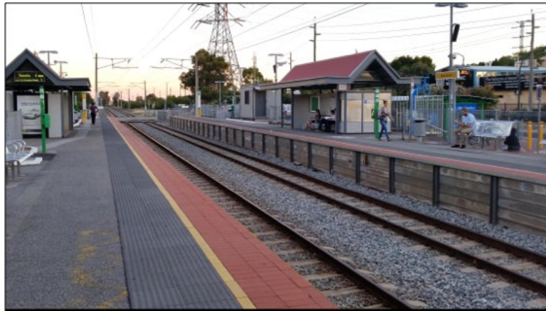
FIGURE 5. Oats Street train station
