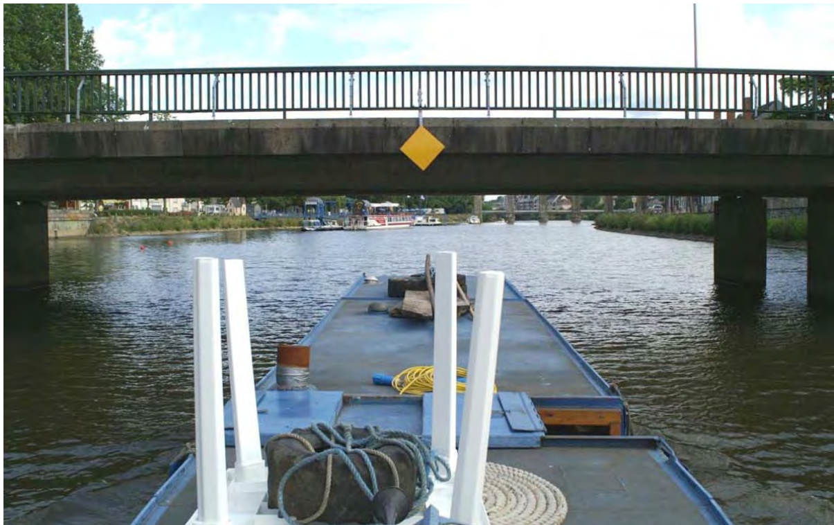
Figure 3.61 Bridge heights must account for rising water levels and different size boats
