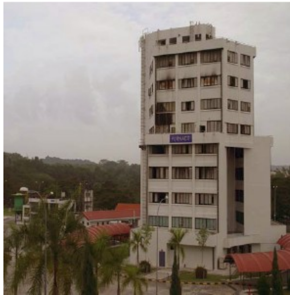
Fire & Rescue Training Tower ('The Furnace') (Figure 14)
