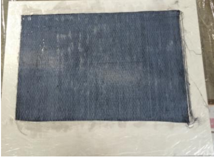
c) Roll epoxy on the top of fiber wrap
