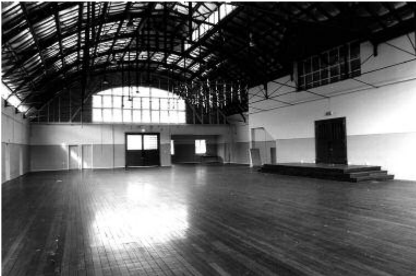
Fig 5 – Perth Drill Hall 2002 interior of drill hall space.
