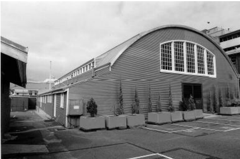
Fig 4 – Perth Drill Hall 2002 from east.
