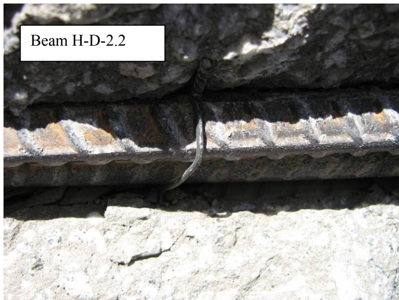
Figure G.3: Steel-Geopolymer Concrete Interface for Beam N-D-2.2 and H-D-2.2
