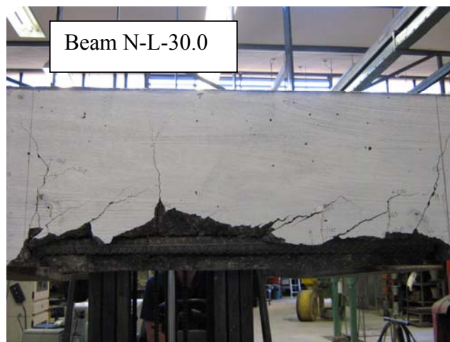
Figure 8.5 : Crack Pattern of Normal Strength Geopolymer Concrete Beams over the Splice Region After Failure (L-Series)
