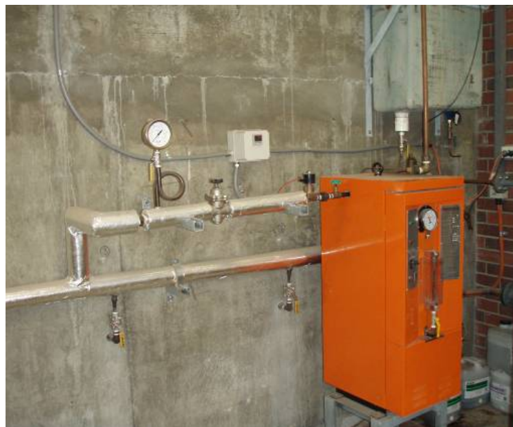
Figure 3.12: Steam boiler system
