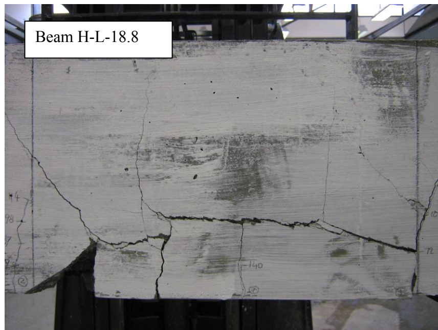
Figure F.5: Crack Pattern for Beam N-L-18.8 and H-L-18.8 (Side View)
