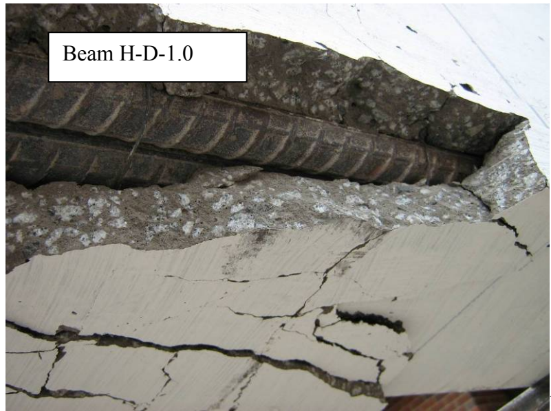
Figure G.1: Steel-Geopolymer Concrete Interface for Beam N-D-1.0 and H-D-1.0
