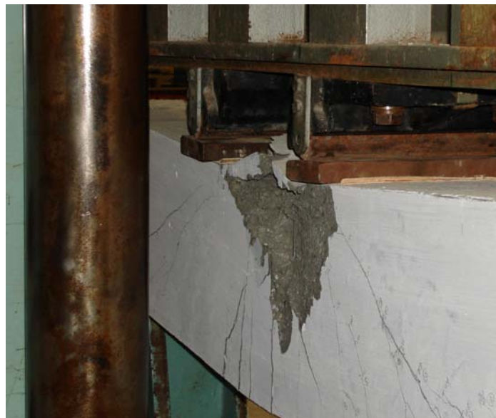
Figure 4.4: Concrete Crushing in Compression Zone for Beam S1-2
