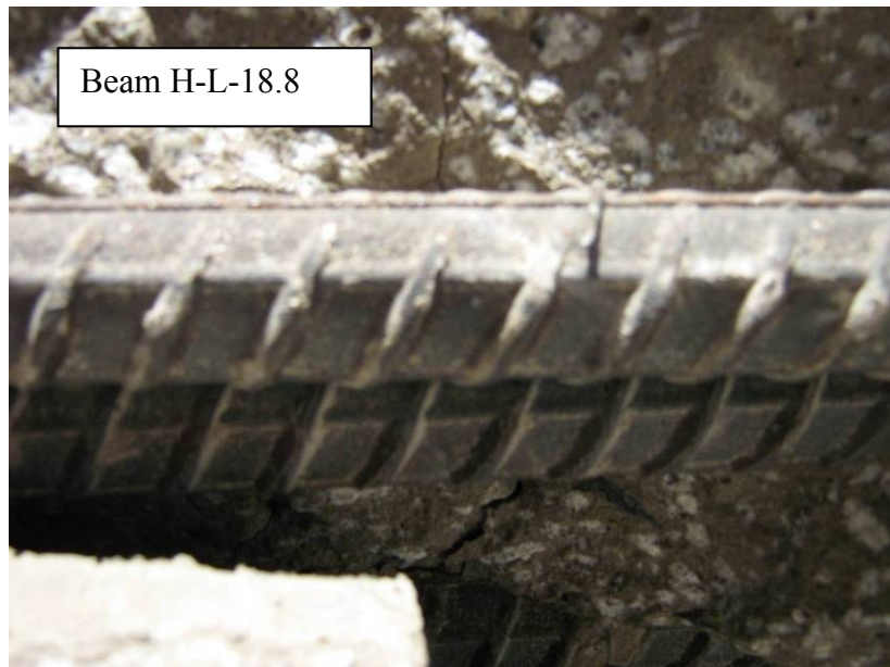
Figure G.5: Steel-Geopolymer Concrete Interface for Beam N-L-18.8 and H-L-18.8
