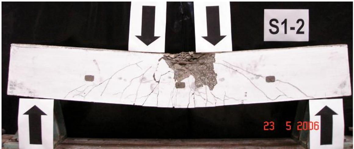
Figure 4.5: Overall Crack Pattern for Beam S1-2 (Front Face)
