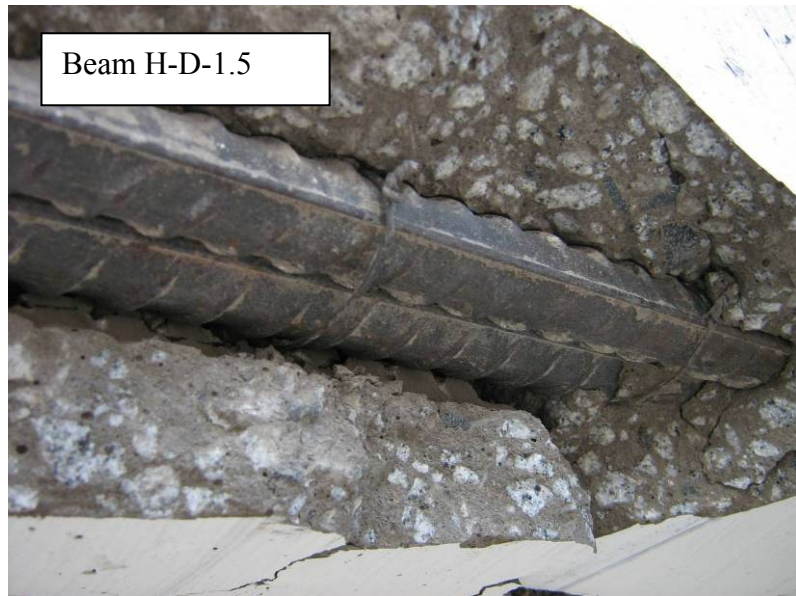
Figure G.2: Steel-Geopolymer Concrete Interface for Beam N-D-1.5 and H-D-1.5
