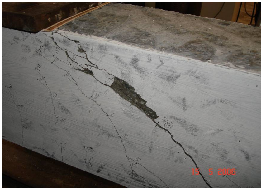
Figure 4.7: Principal Diagonal Crack Near Loading Point for Beam S1-3
