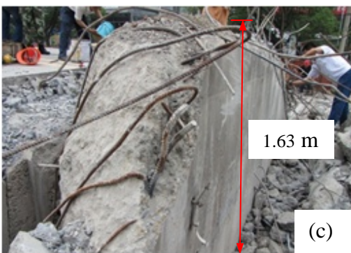
Fig. 6. Hongqi Viaduct after collapse: (a) overview, (b) collapsed slabs, (c) remaining pier (#109) and (d) pier #101
