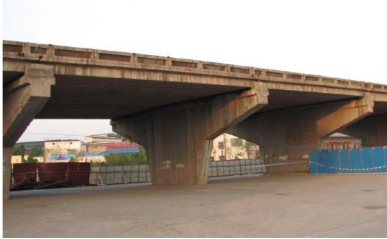
Fig.1. Typical view of Hongqi Viaduct (before collapse)
