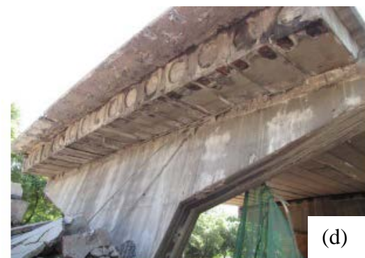
Fig. 6. Hongqi Viaduct after collapse: (a) overview, (b) collapsed slabs, (c) remaining pier (#109) and (d) pier #101
