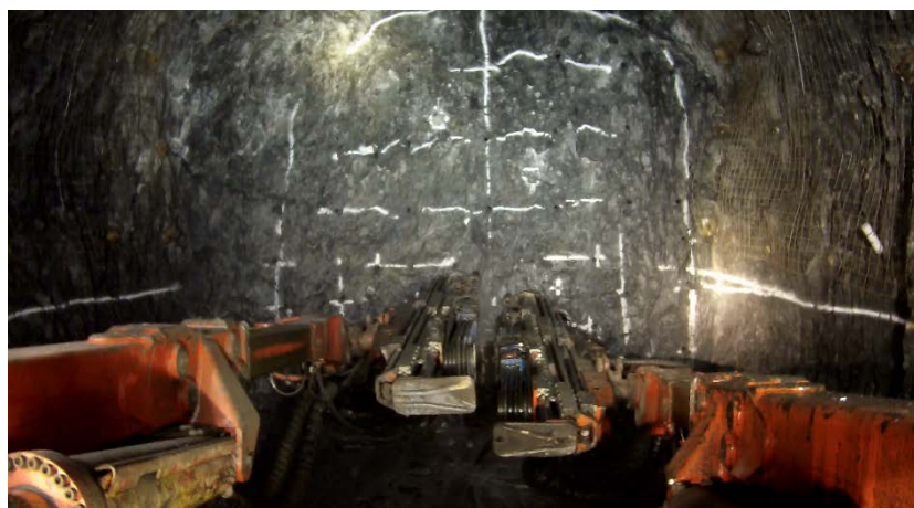
Figure 9: Two booms drilling simultaneously
