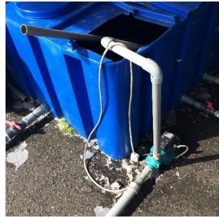
Figure 3.5: Centrifugal pump to transfer raw septage from the storage tank to the feed tank
