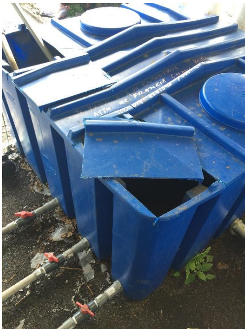
Figure 3.6: 250-gallon distribution tank
