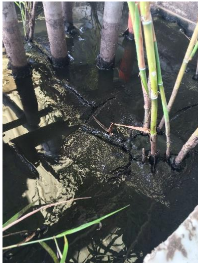
Figure 5.21: Cracks formed via the mechanical vibration of the reed stem caused by the strong wind
