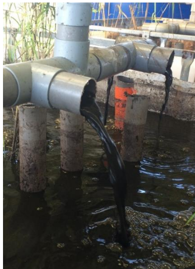
Figure 3.13: Distribution device during loading
