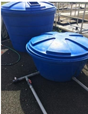
Figure 3.2: 400-gallon and 100-gallon storage tanks
