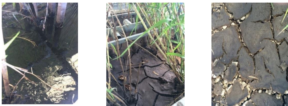
Figure 5.17: (Left) The slurry with high water content accumulated on the surface of the wetland bed right after loading. (Center) Some cracks formed on the top surface of sludge deposit layer during resting period. (Right) The large cracks exposed the gravel layer after the extended resting period
