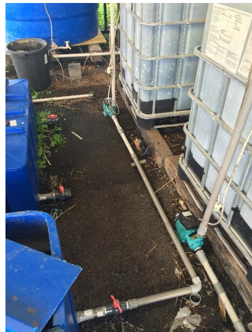
Figure 3.7: Pipe connection between the distribution tank and the centrifugal pumps
