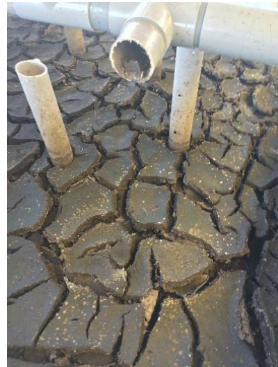
Figure 5.22: Cracks formed in the controlled bed during resting period
