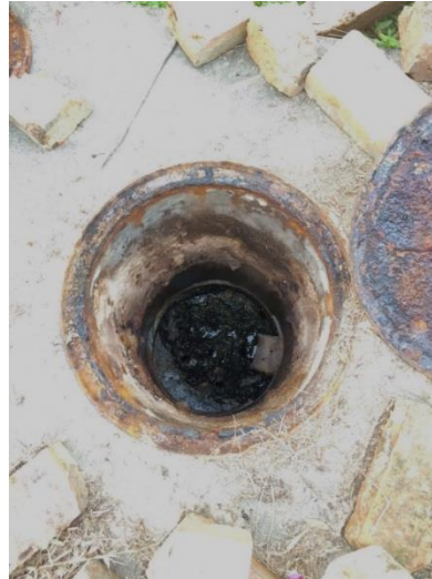
Figure 1.1: Septic tank with excessive sludge
