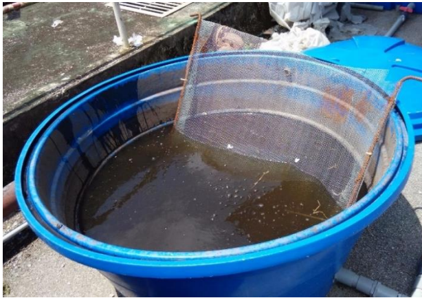
Figure 3.4: Secondary screening process in the 100-gallon storage tank before the raw septage was discharged to the feed tank
