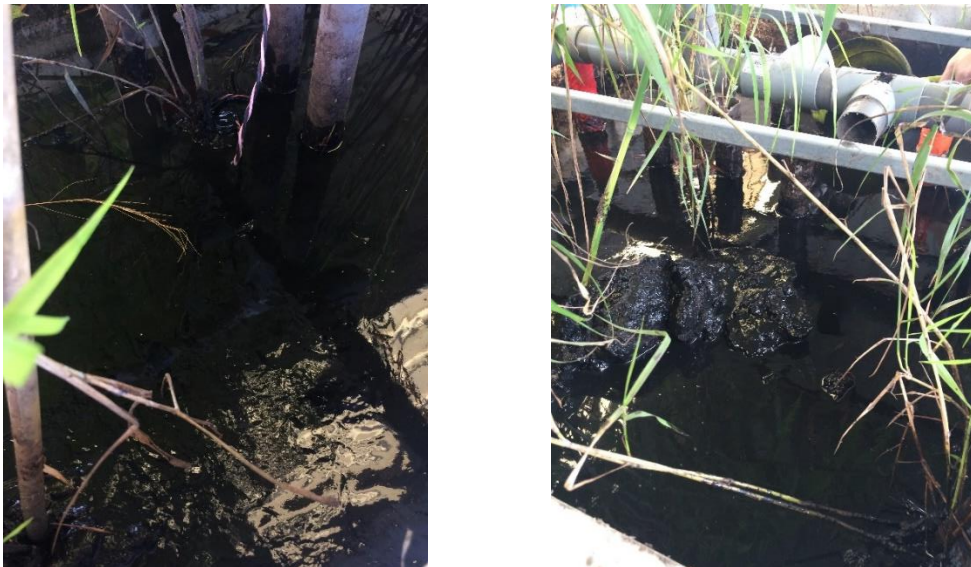
Figure 6.20: Stagnant raw septage at the wetland surface during later stage of treatment
