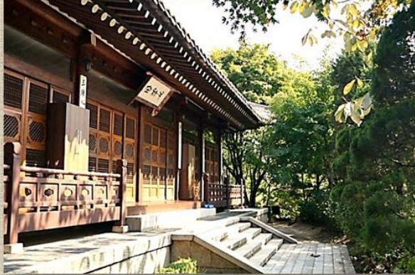
The front entrance of Sam Cheong Gak Restaurant
