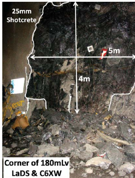
Figure 8.36. Photograph of 20m 2 of heavy spall damage of thinly shotcreted development on 180mLv drive LaDS after 180mLv mass firing.
