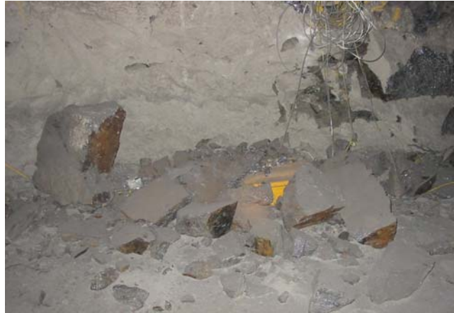
Figure A4.21. Data acquisition system buried by pillar spall on the 220mLv level at BHP Cannington Mine.
