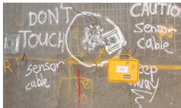
Figure A4.20. Blast monitoring equipment attached to weld-mesh using utility hooks at the BHP Cannington Mine.
