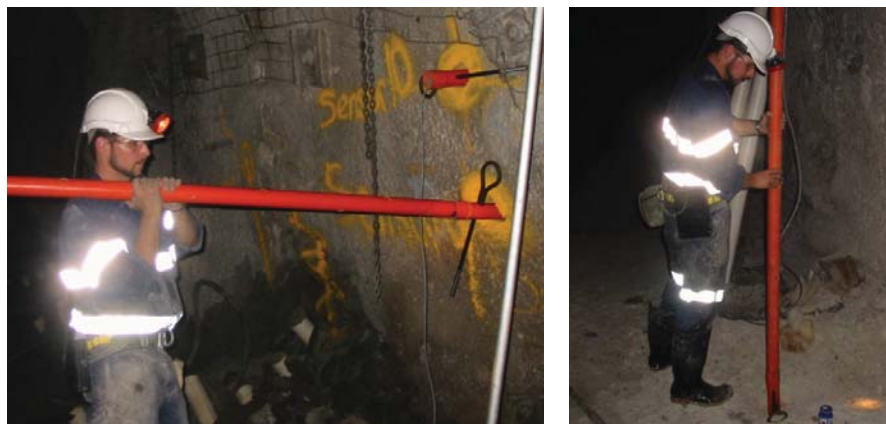
Figure 4.3. Installation of tri-axial transducers in the hangingwall (left) and footwall (right) of Kanowna Belle Gold Mine stope dB10-38T.
