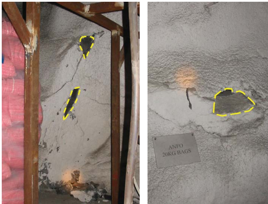
Figure 8.22. Pictures of spalled shotcrete in the 240mLv explosives magazine occurring with the mass blast or main rings firing of stope 22gC6HL.
