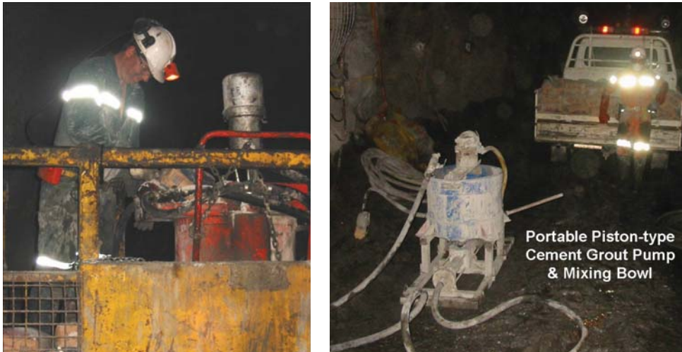
Figure A4.22. I.T. mounted grouting basket used at the Kanowna Belle Gold Mine (left) and portable piston pump and mixing bowl used in sensor installation at the Cannington Mine (right).
