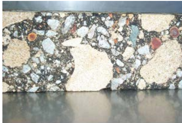
Figure 1. Example of a foamed bitumen beam section extracted from the pavement trial
