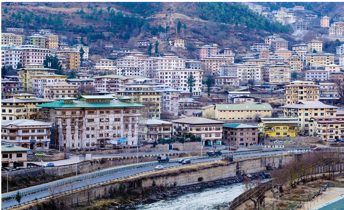
Figure 6-1 Typical masonry infilled RC buildings in Thimphu, Bhutan.
