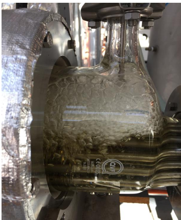
Figure 4: MEG Distillation Column Reboiler
