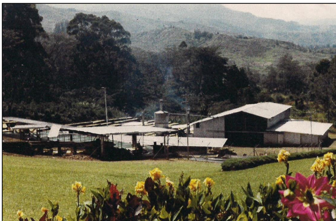
Plate 4.1: A coffee factory complex at Nomba Coffee Plantation, Upper Asaro, EHP in 1979 (Source: John Fowke).
