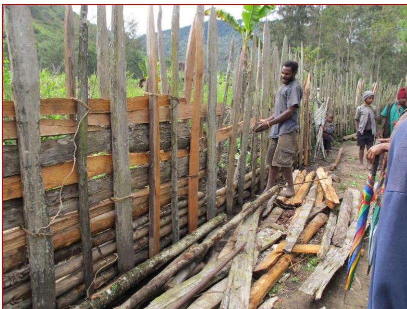
Plate 5.1: Garden fence being constructed.
