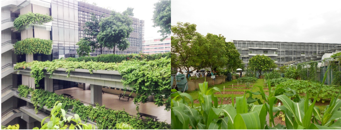
Figure 7-16: KTP hospital, multilevel gardens and green roof.
