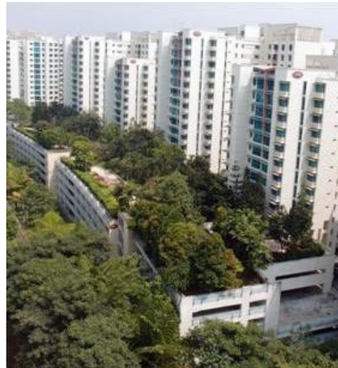
Figure 7-18: Integrated MSCP roof garden
