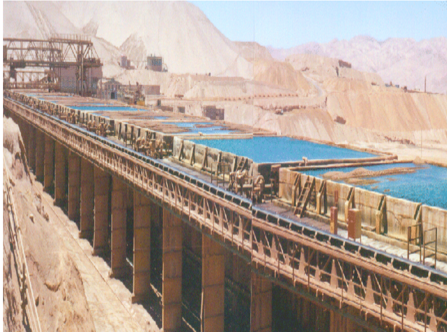
Figure 2.14 Vat leaching of copper at Mantos Blancos, Chile, 1995 (Source: INNOVAT Limited)
