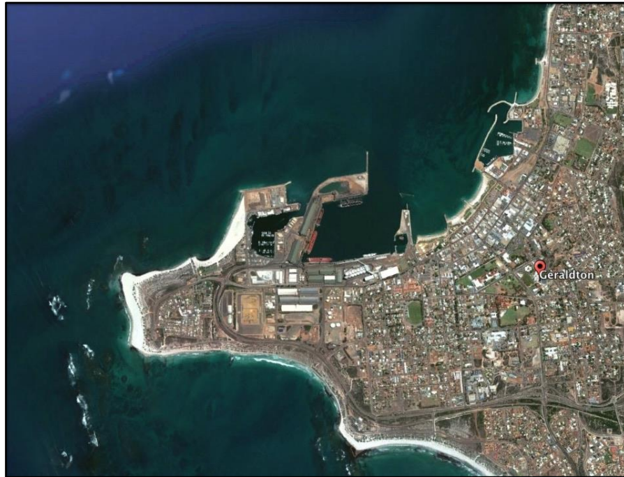
Figure 2: Geraldton coastal infrastructure. Source: Google (2016).
