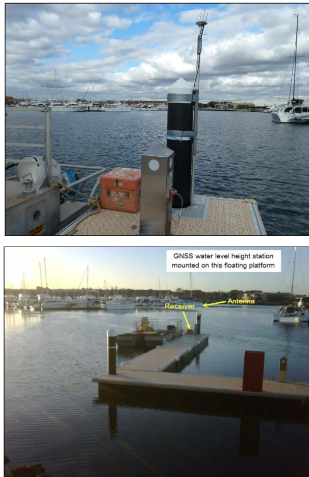
Figure 3.1: GNSS antenna and receiver for the nearshore study. (Top) Installation of the GNSS antenna and receiver. (Bottom) Pontoon used to install the GNSS antenna and receiver at Hillarys Boat Harbour, Western Australia (Kennedy, 2011)
