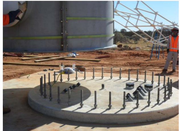
Fig. 4 An ASKAP antenna pedestal being lowered onto the foundation. The “upstand” in the centre of the foundation is 3m diameter x 150mm high
