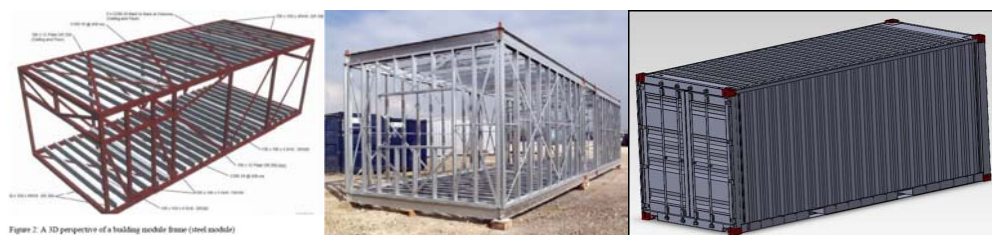
Figure 2: (L) Modular steel building [31], (M) Light steel framed module [12], (R) Shipping container [26]
