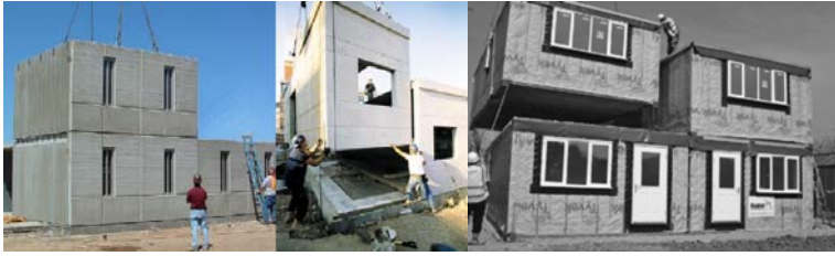
Figure 3: (L) Precast concrete modules [17]; (R) Timber frame modules [4]
