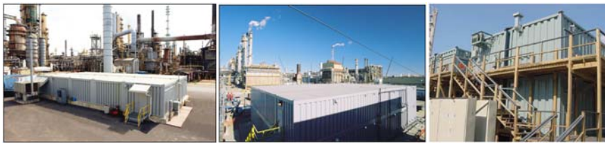
Figure 7. (L) One storey BRM building [96], (M) Two storey BRM building [96], (R) Stacked BRPB complex [97]
