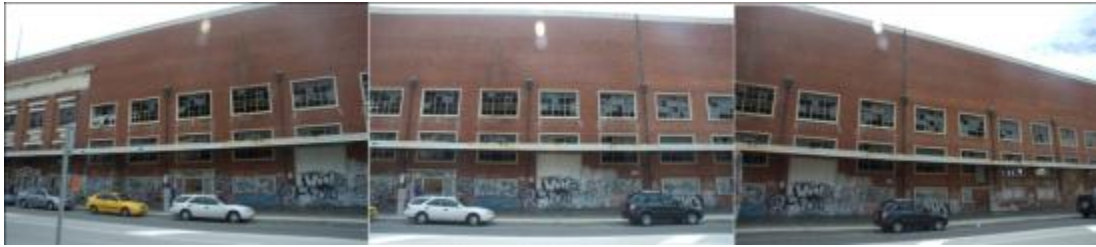
Figure 6.1: Wool Stores building. (Source: Honni Mansell)
