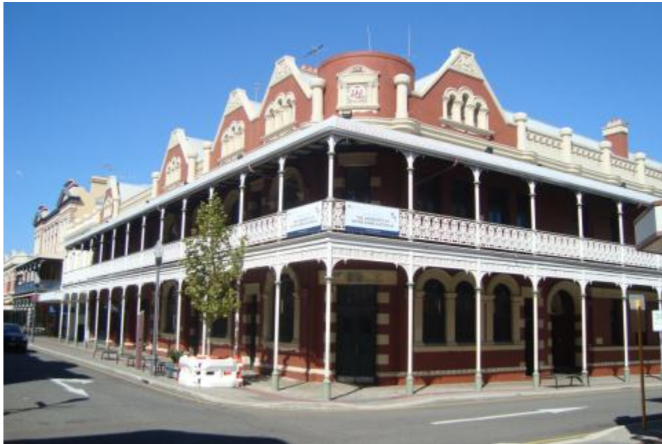
Figure 4.11 The P&O Hotel on the corner of High Street and Mouat Street.
