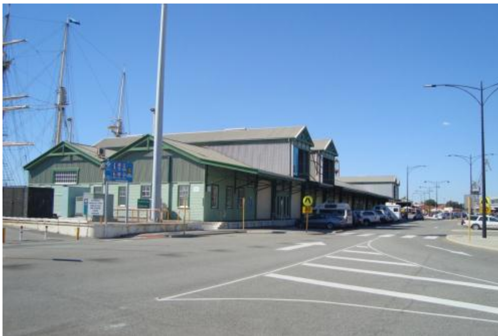
Figure 5.4 B-Shed. (In the process of being adaptively recreated as a café.)
