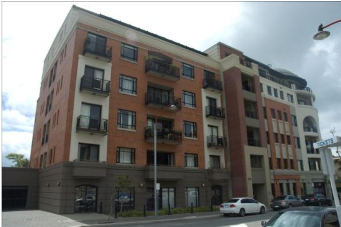
Figure 6.11 VQA stage one apartments (opposite Clancy's fish pub).
