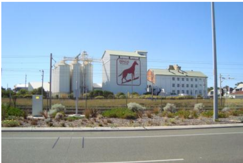
Figure 1.4: The Dingo Flour Mill (still in operation).
