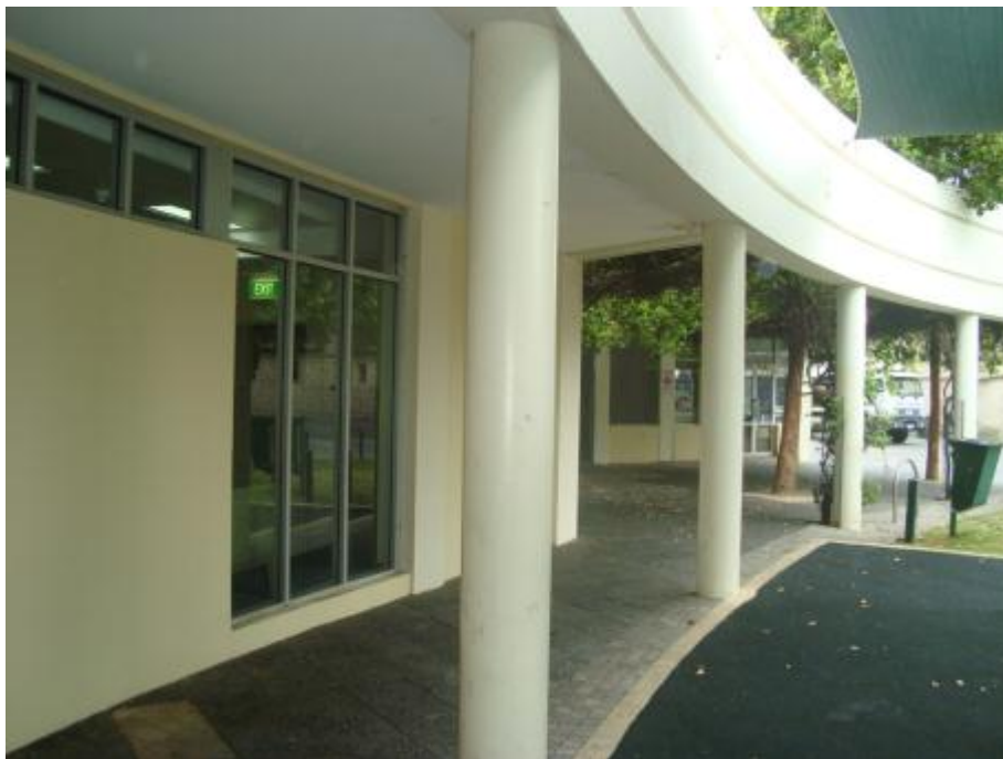
Figure 7.10 White pillars outside the local history section of the Fremantle library.
