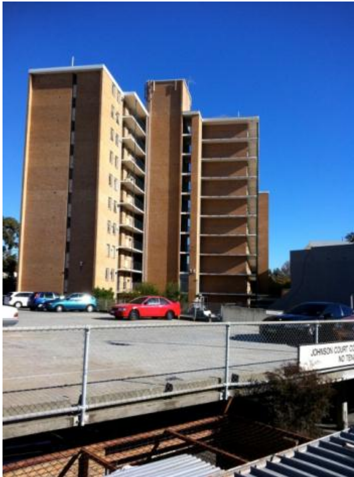
Figure 6.3 Johnson Court flats (built in the 1960s and considered to be an example of ‘bad planning’ and ‘architectural vandalism’ (Dowson 2004b)).
