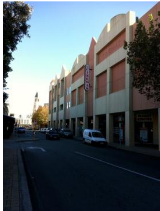
Figure 3.15 Queensgate building adjacent to Kings Square
