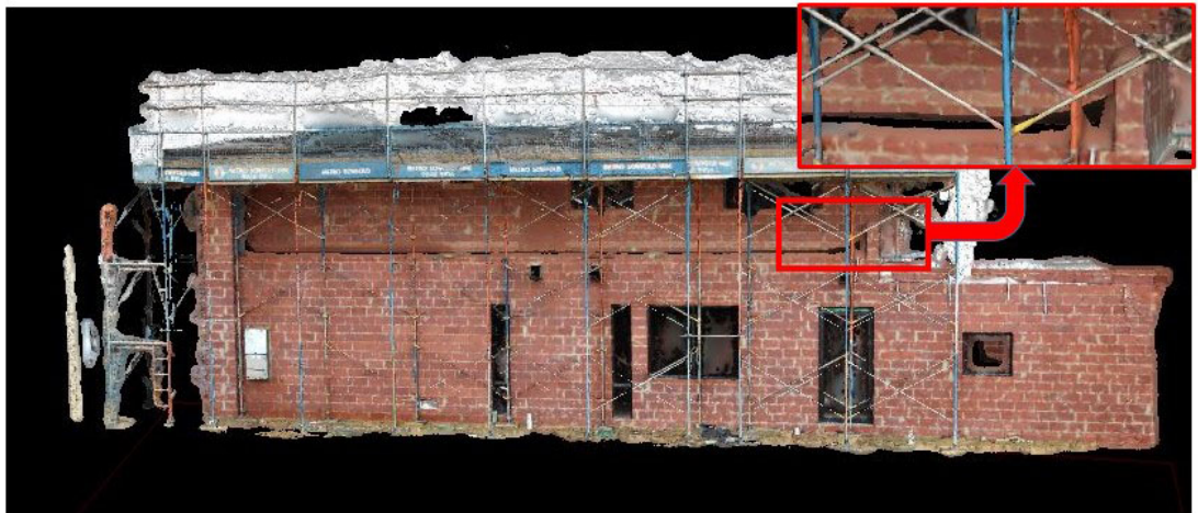
Figure 4.9. Reconstructed scaffolding with photos from a commercial DSLR camera
