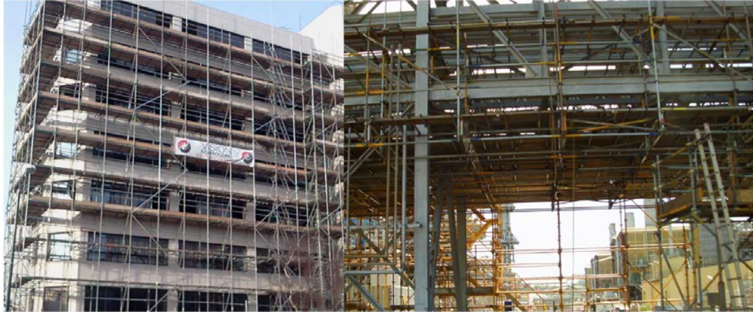
Figure 6.3. The scaffolding and backgrounds with similar appearance
