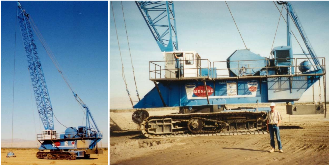
Figure 2-110: Lampson crane modified by dynamic compaction
