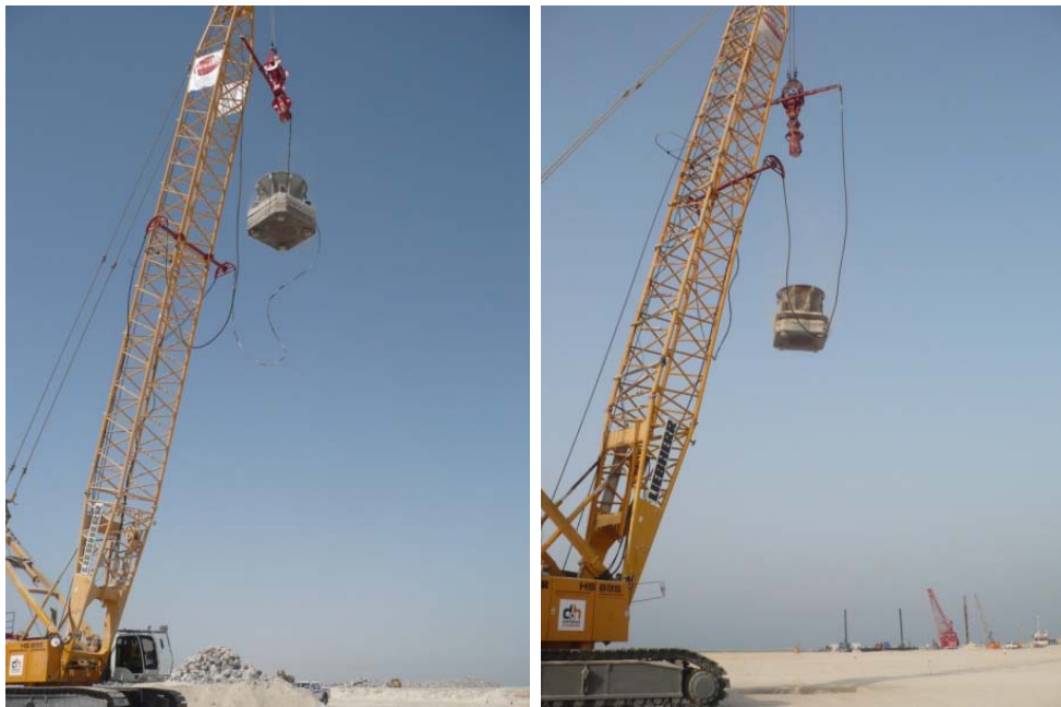
Figure 3-115: Free fall drop of a 35 ton pounder using MARS technology
