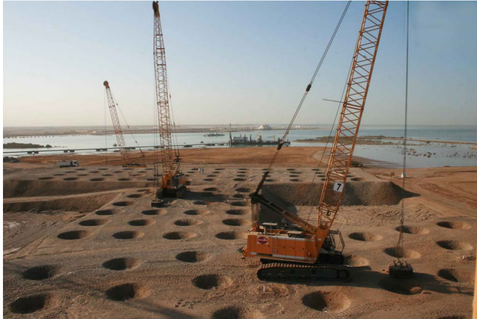
Figure 3-49: Dynamic Surcharging in KAUST
