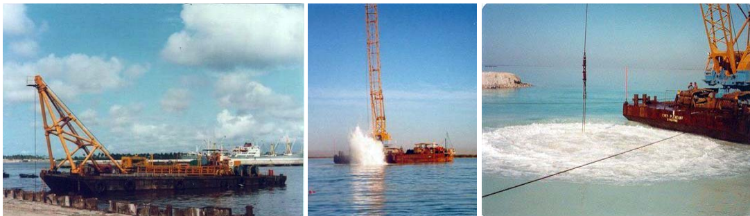
Figure 2-195: Dynamic compaction at Lagos dry docks, Nigeria
