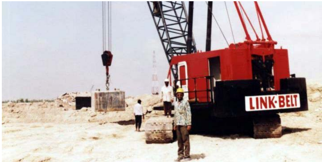
Figure 2-112: Reinforced concrete pounder encased in a steel box
