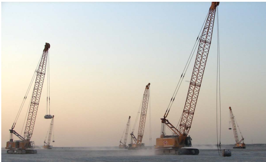
Figure 3-61: Implementation of 11 special cranes for DC (not all shown in this photograph)
