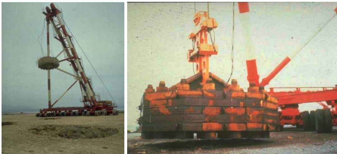
Figure 2-4: The Giga Machine holds the world record for lifting a 172 ton poulder at Nice International Airport dynamic compaction project (Communication Department of Menard, 2007)
