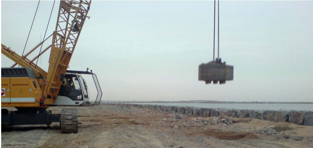
Figure 3-92: Application of dynamic compaction at the vicinity of slope armour protection
