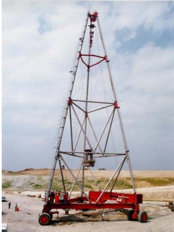
Figure 2-107: Dynamic compaction using the Menard tripod
