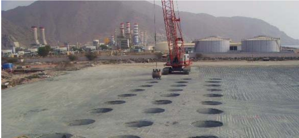
Figure 3-247: Dynamic Compaction at Fujairah Desalination Plant
