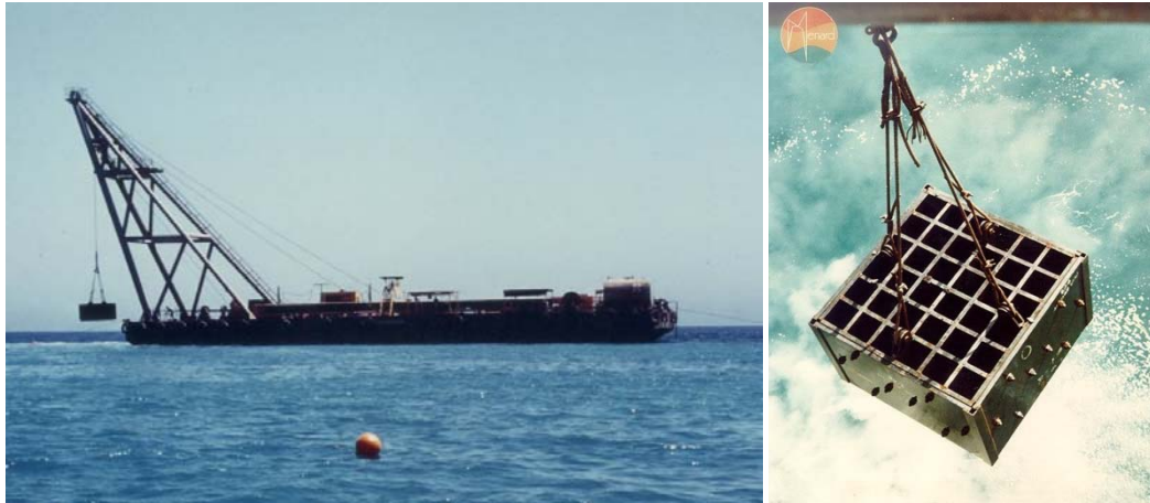
Figure 2-194: Offshore DC at Kuwait Naval Base using a 32 t specially designed pounder
