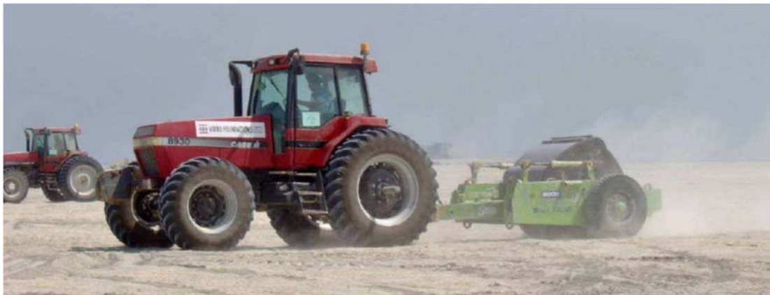
Figure 2-116: Impact roller compaction
