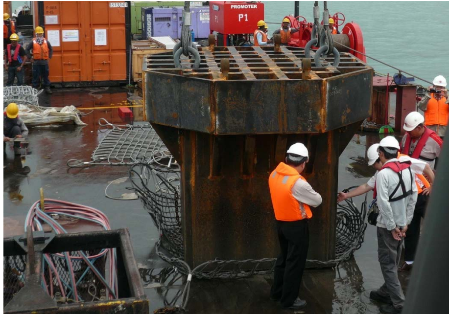
Figure 3-229: Marine DR (bottom side) - DC (top side) pounder
