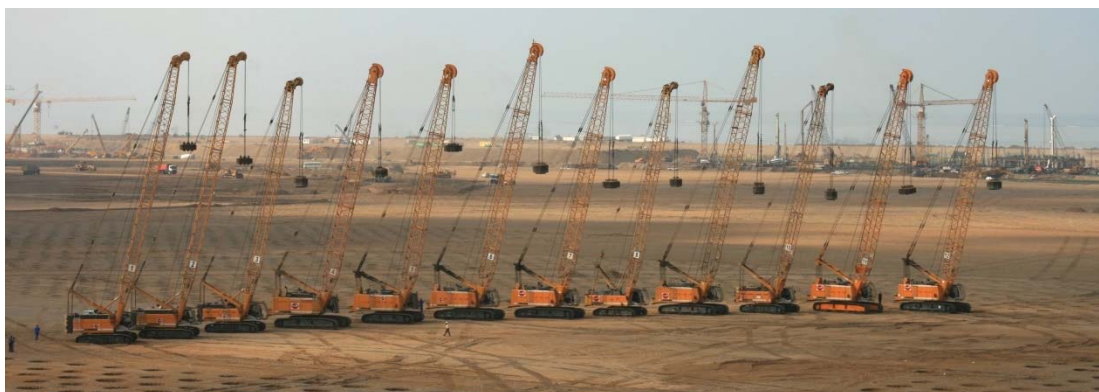
Figure 3-51: Utilisation of 13 DC-DR rigs in two shifts (photograph taken from the 13 th rig)
