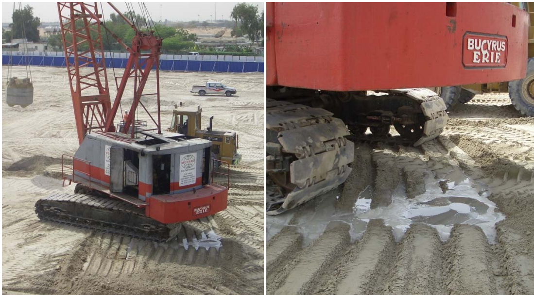
Figure 3-144: Release of excess pore water pressure in the form of sand boiling
