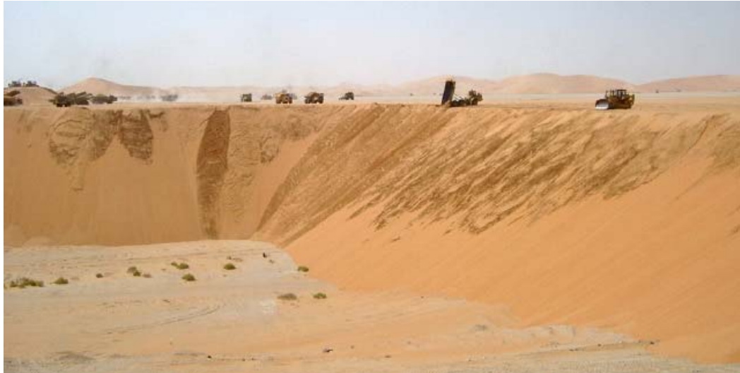
Figure 3-21: Grand size cutting and dump filling of dune sands for the construction of the second phase of Al Quo'a Township.
