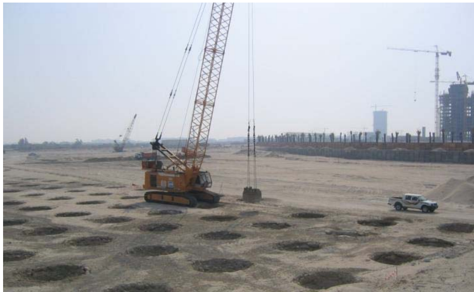
Figure 2-109: Dynamic compaction using 25 ton pounder
