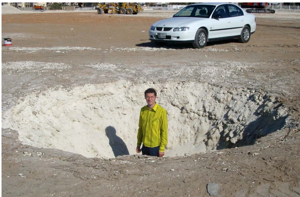
Figure 3-8: Typical crater size and depth in the deep treatment areas of Abu Dhabi New Corniche
