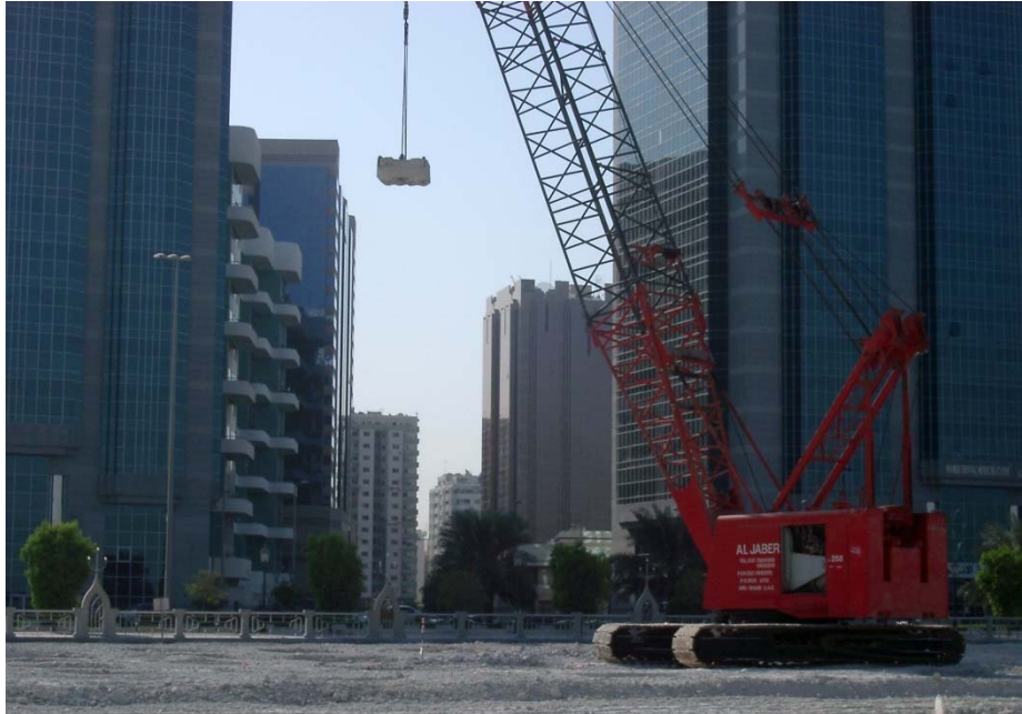
Figure 3-10: Application of dynamic compaction in front of Abu Dhabi skyline
