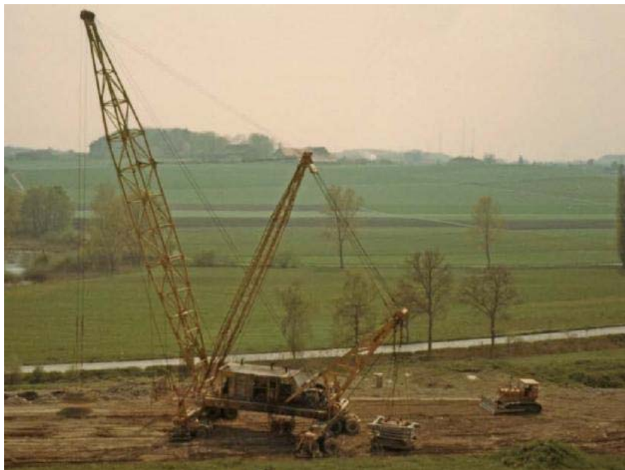
Figure 2-106: Dynamic compaction using 1,600 tm mega machine (Communication Department of Menard, 2007)
