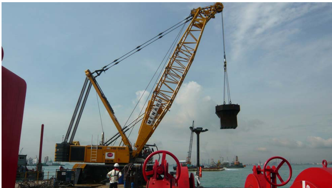
Figure 3-230: Marine pounder being utilised for dynamic replacement
