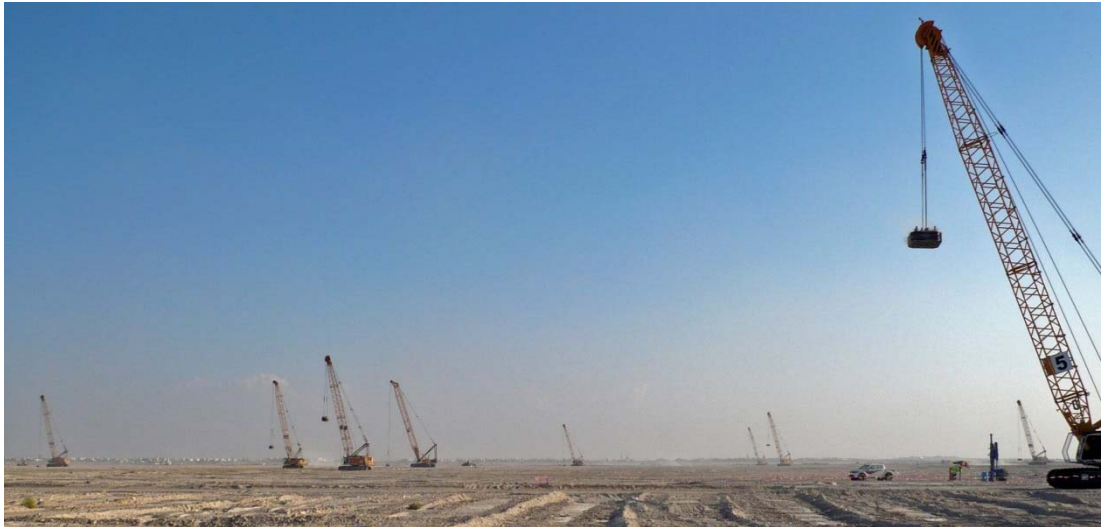
Figure 3-4: Treatment of 4.84 million m 2 of loose sands at Al Falah Community.
