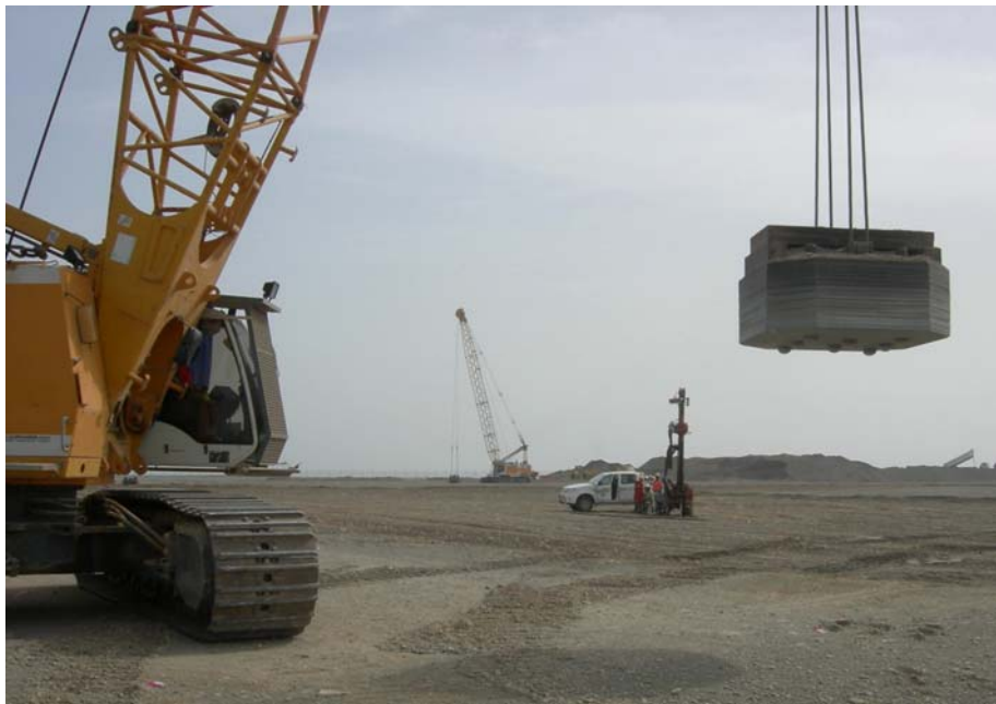
Figure 3-254: Application of dynamic compaction at Medina A'Zarqa using a 23 t pounder
