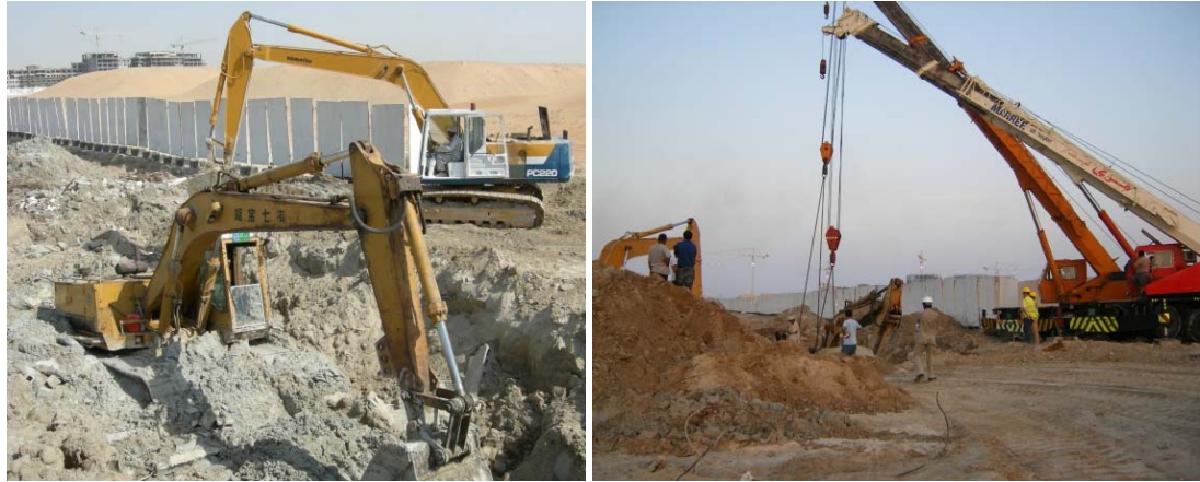
Figure 3-142: Construction equipment sinking into the ground due to poor ground conditions
