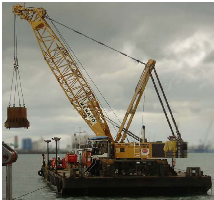
Figure 3-231: Marine pounder used for dynamic compaction
