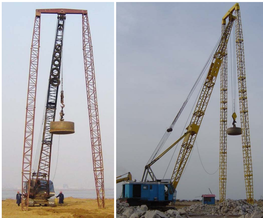
Figure 2-111: Dynamic compaction in China using cranes that have been modified into tripods
