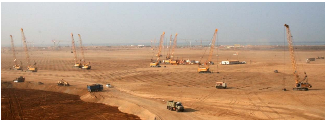
Figure 3-3: Application of DC and DR at KAUST using 13 (9 shown in the photograph) DC-DR rigs working in two shifts per day.
