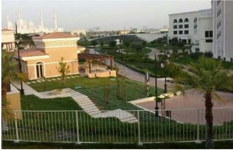
Figure 3-152: Completed chalets at Abu Dhabi Ritz-Carlton Hotel
