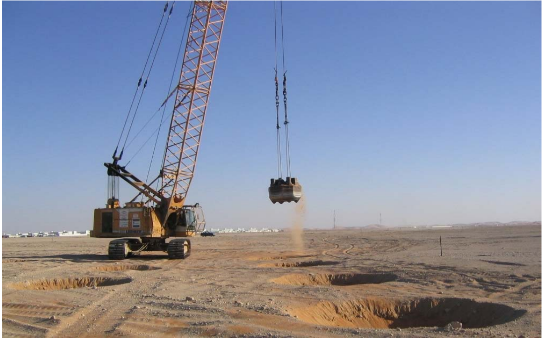
Figure 3-26: DC rig for lifting 25 ton pounders at Al Quo'a
