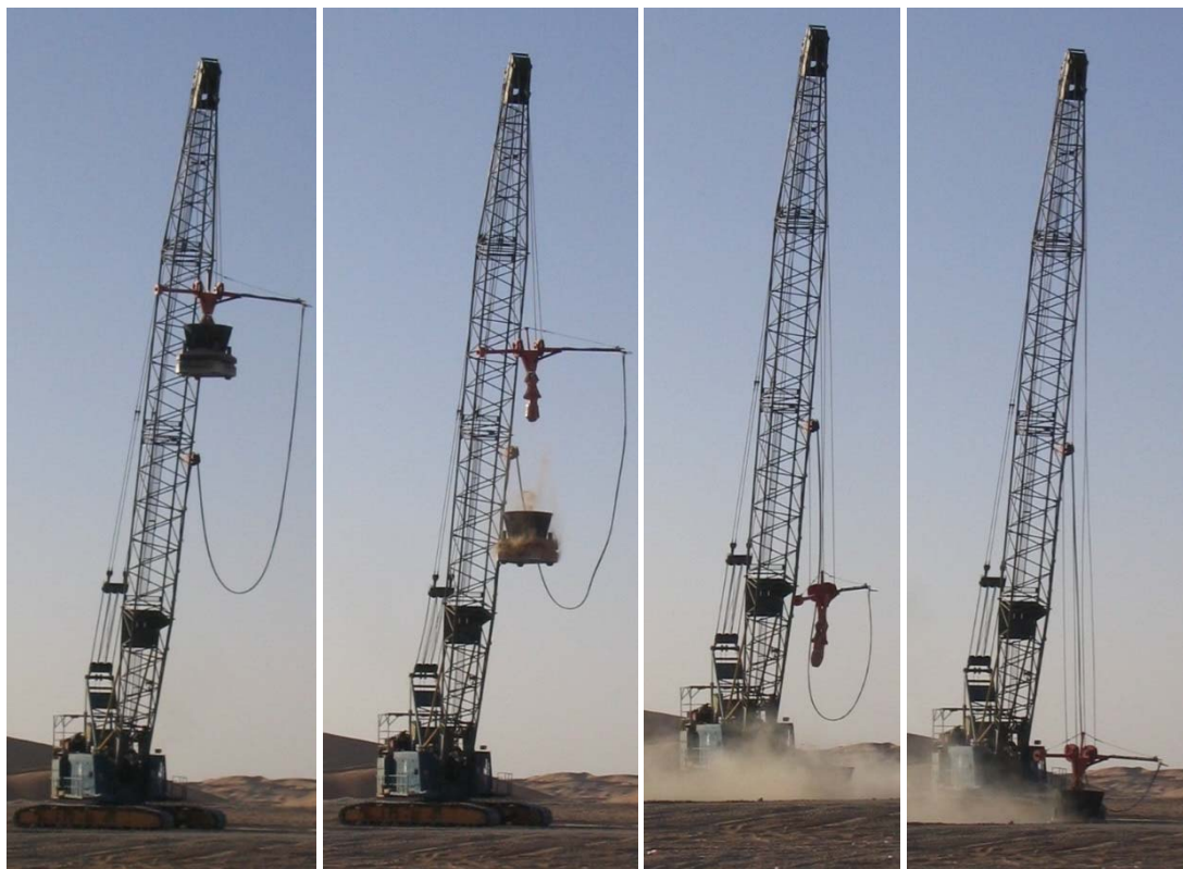
Figure 3-23: Free fall of 35 ton pounder using MARS
