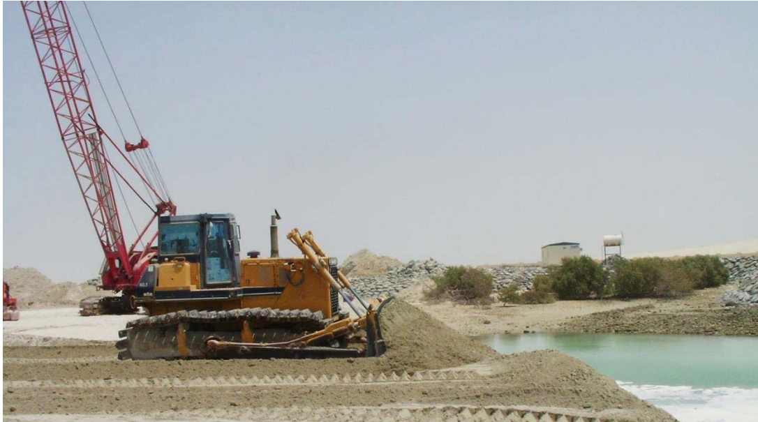
Figure 3-169: Reclamation by dumping sand and pushing it into the sea
