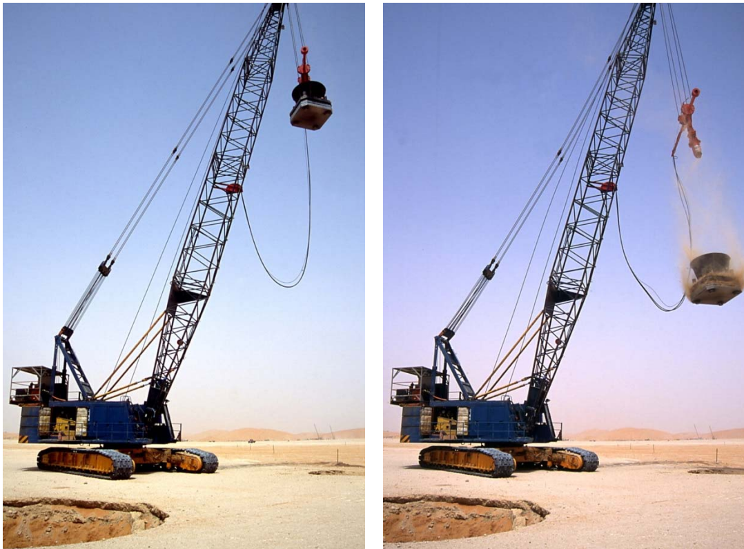
Figure 3-2: First application of MARS pounder release and reconnect mechanism in the world
