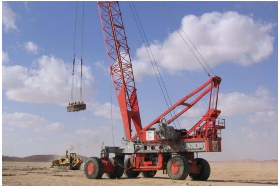
Figure 2-105: Dynamic compaction using the 700 tm rig
