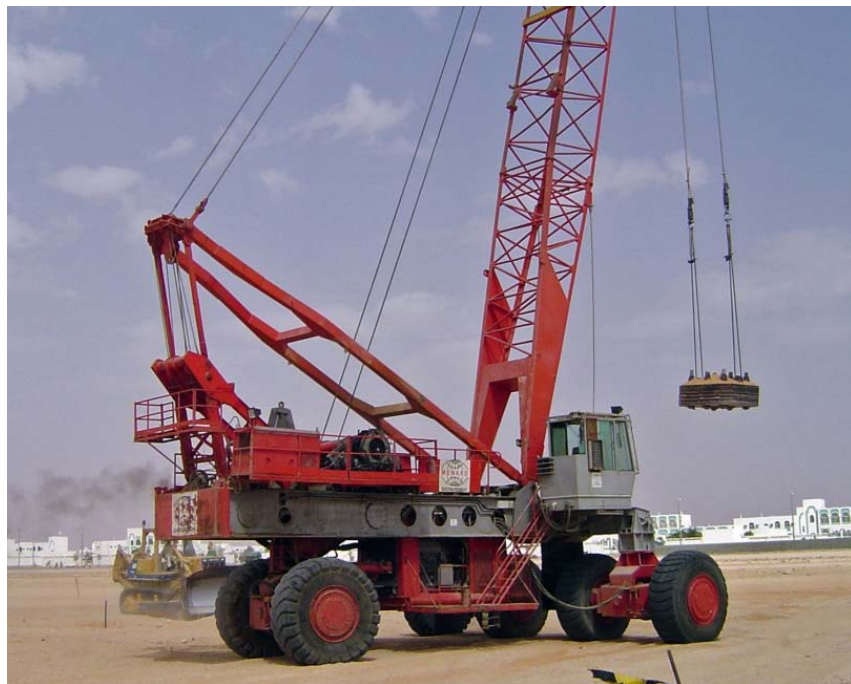
Figure 3-27: Menard 700 tm rig at Al Quo'a
