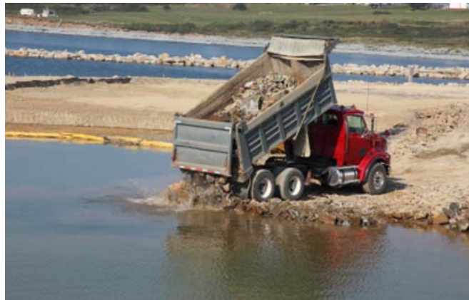
Figure 2-188: Dump truck tipping fill into the sea
