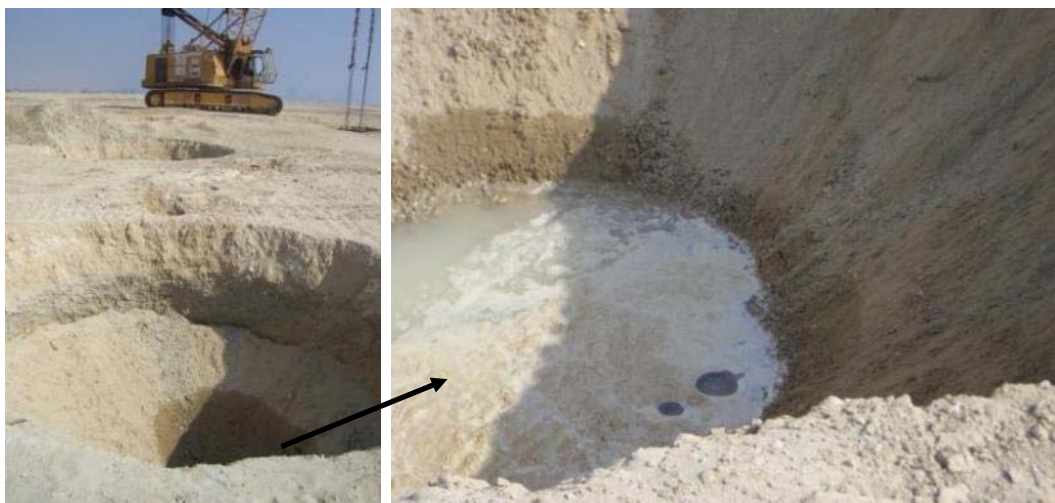
Figure 2-24: Appearance of water fountains from the fissures due to dynamic compaction
