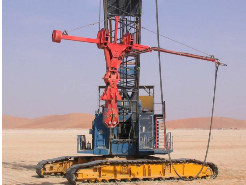
Figure 3-28: 250 ton rig for lifting the 35 ton pounder using MARS
