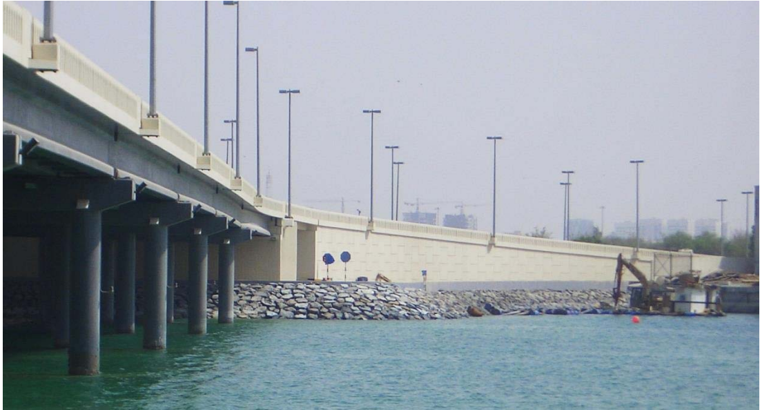
Figure 3-178: Abu Dhabi – Reem Island Causeway after completion
