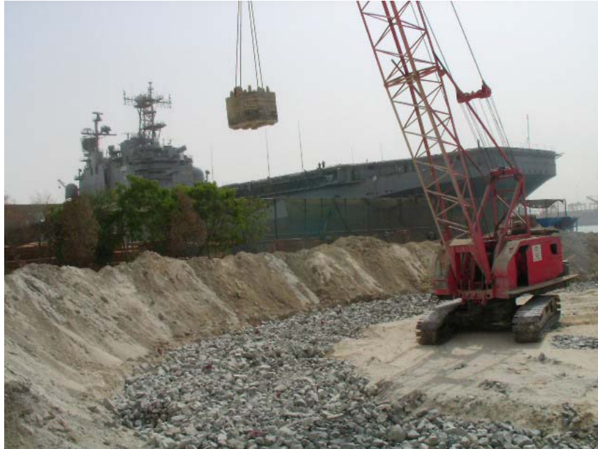
Figure 3-223: Dynamic compaction of the shear ring
