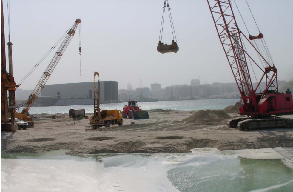
Figure 3-170: Application of dynamic compaction at Reem Island Causeway
