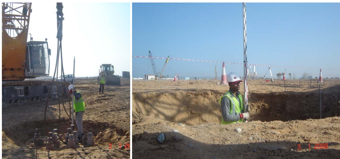
Figure 3-95: Measurement of crater depth in the heave and penetration test
