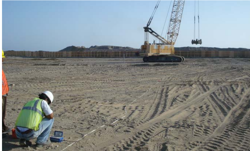
Figure 3-255: Dynamic compaction vibration monitoring at Medina A'Zarqa
