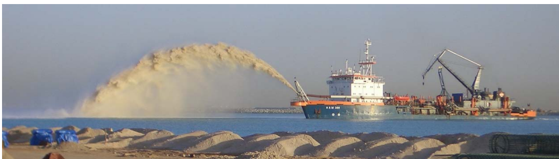
Figure 3-192: Reclamation by rainbow discharge at Palm Jumeira
