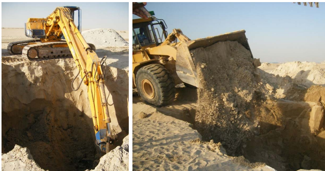
(a) (b) Figure 3-157: (a) Pre-excitation, (b) backfilling with sand
