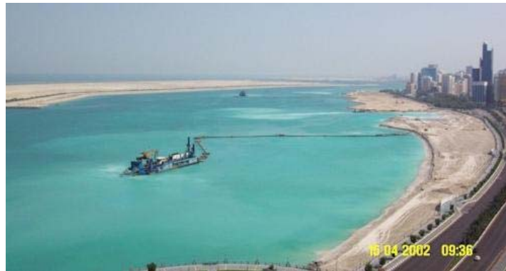
Figure 3-7: Reclamation of New Corniche by pipeline discharged hydraulic fill
