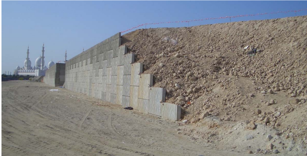
Figure 3-149: Construction of hills supported by MSE walls on one side
