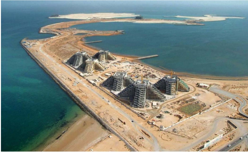
Figure 3-112: Marjan Island road after completion of dynamic compaction works
