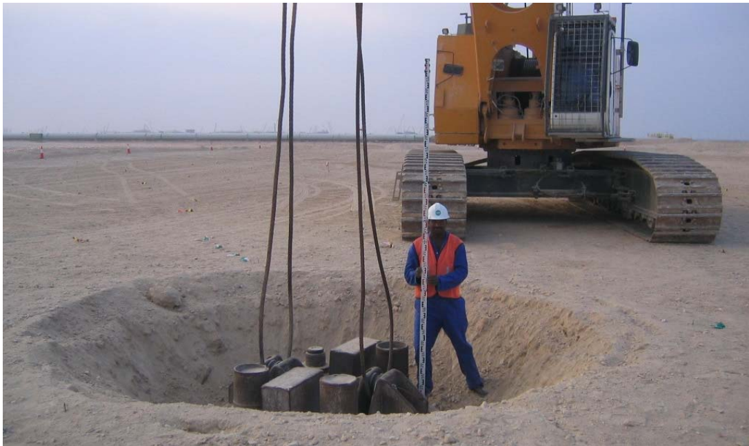
Figure 2-148: heave and penetration test
