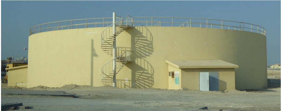
Figure 3-210: Tank A-A after construction
