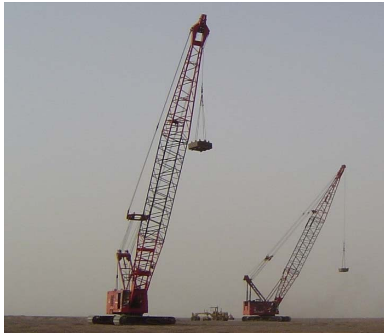
Figure 3-25: DC rig for lifting 15 ton poulders at Al Quo'a
