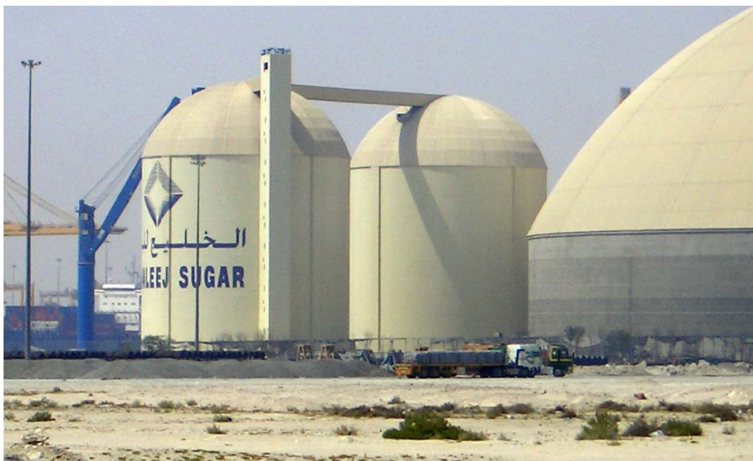
Figure 3-227: Al Khaleej raw sugar silos after completion of construction
