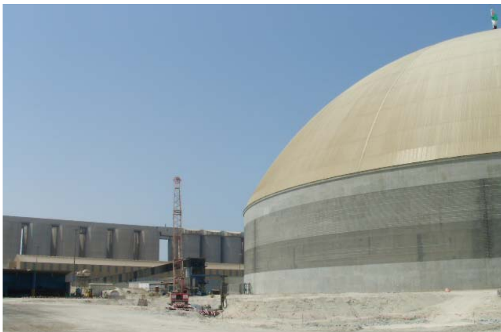
Figure 3-224: Dynamic replacement next to an existing concrete silo
