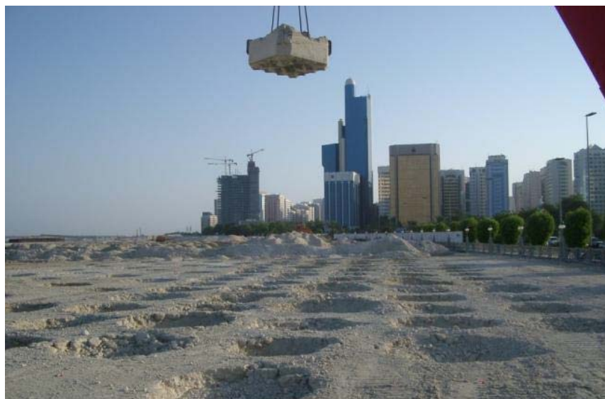
Figure 2-53: Application of Dynamic Compaction in a grid
