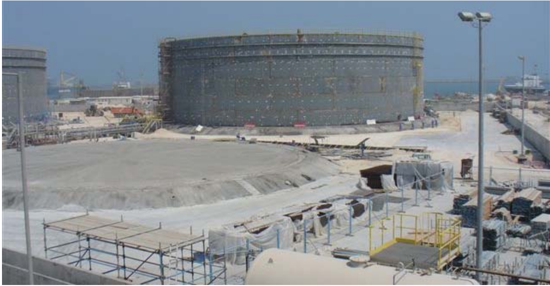
Figure 3-191: HFO tanks under construction
