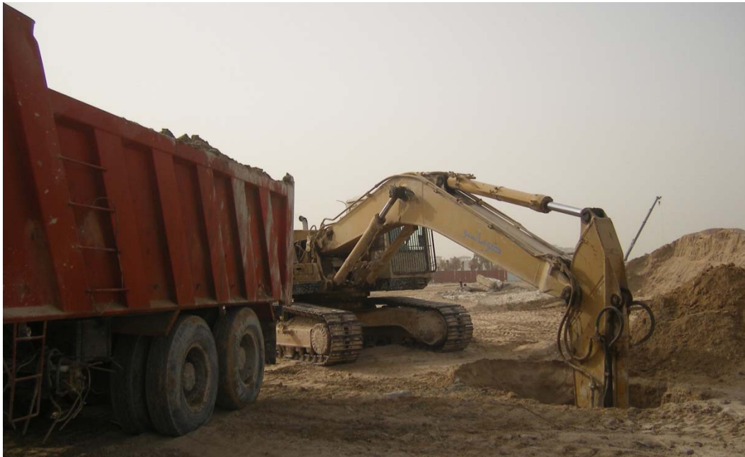
Figure 3-143: Pre-excavation of DR prints
