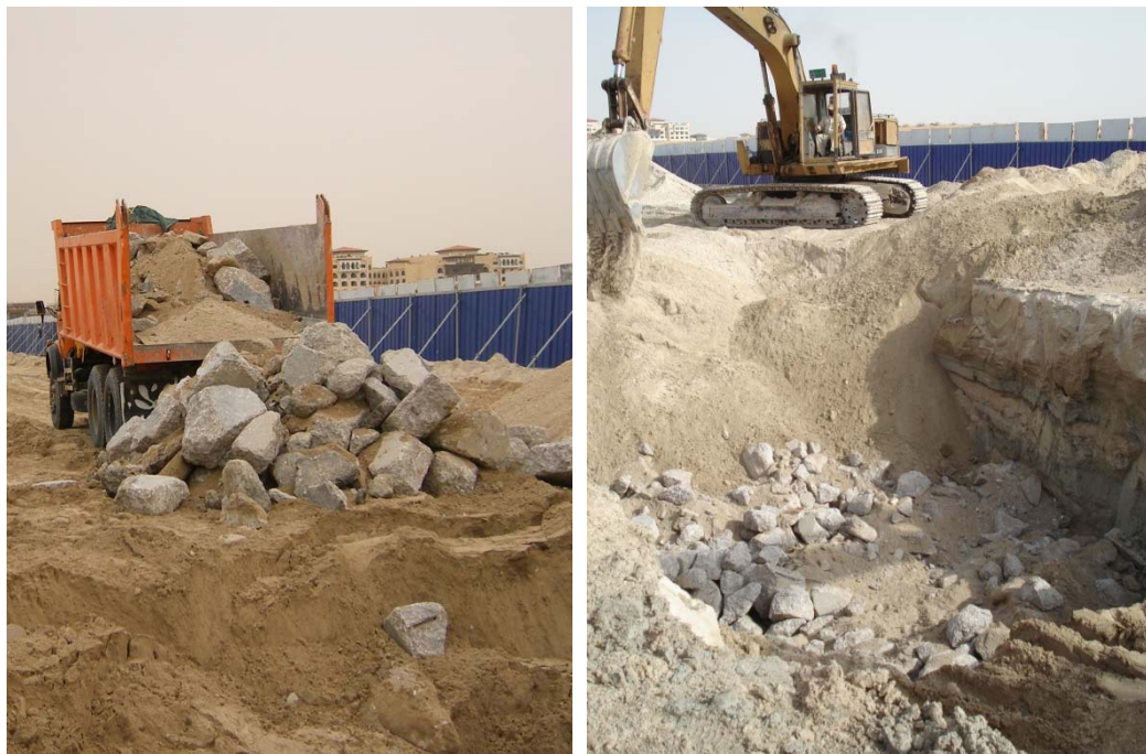
Figure 3-146: Backfilling of the lower part of the trenches beneath the wall with demolished concrete debris
