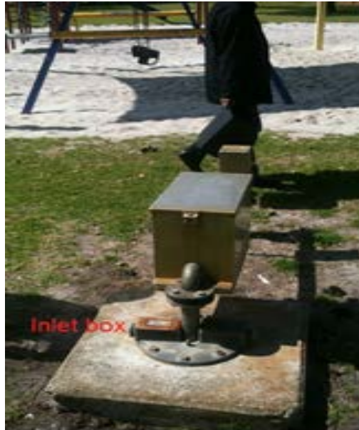
Figure 3:18- Common boreholes with inlet box
