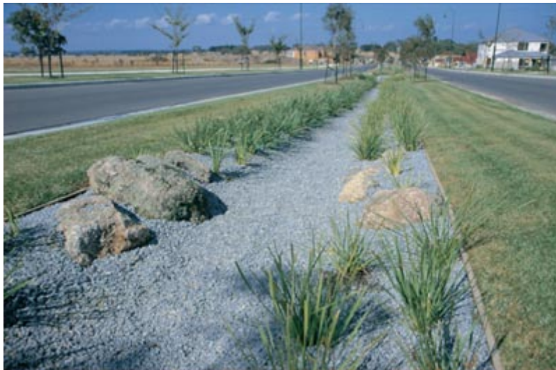
Figure 7:6 - Infiltration trench filled with appropriate sized gravel
