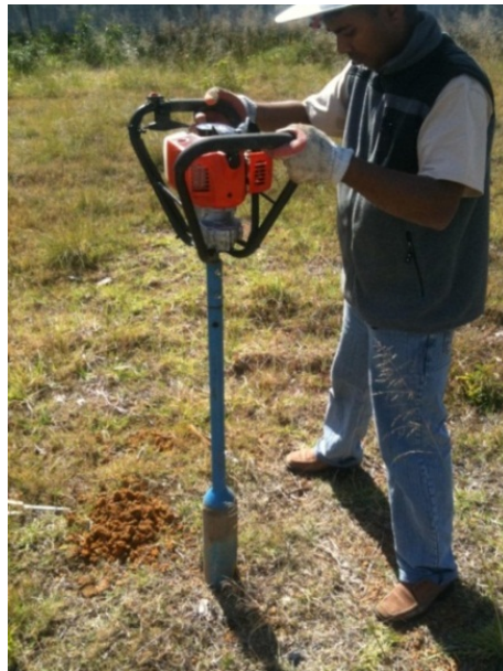
Figure 3:10 - Machine auger being used for excavation
