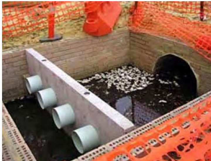
Figure 7:22 –Litter and Sediment trap Source – SWMM-WA
