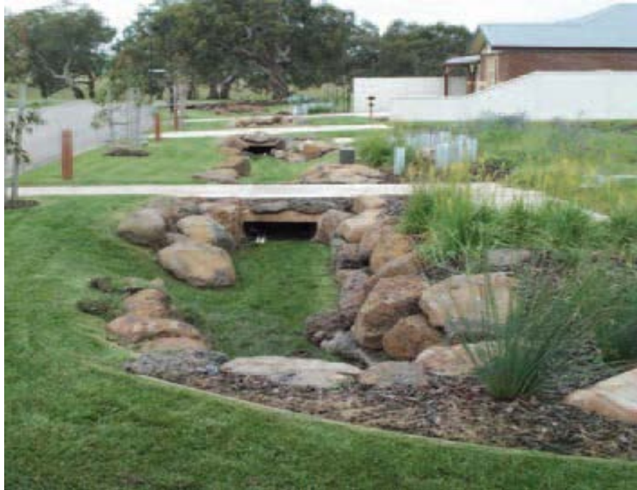
Figure 7:10 – Buffer Zone or Filter Strips
