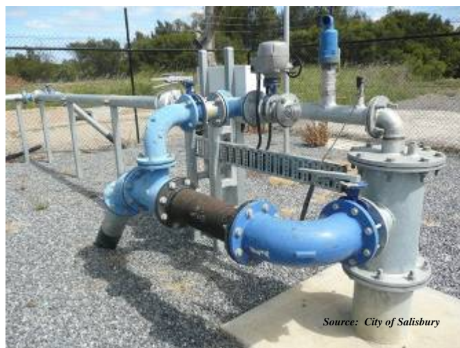
Figure 7:21 –Managed Aquifer Recharge (Source: City of Salisbury)
