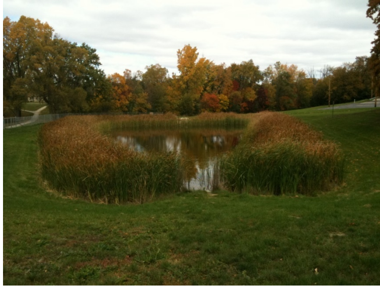
Figure 7:18 –Wet Basin Source – WSUD Engineering Guidelines
