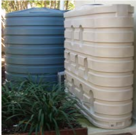
Figure 7:20 –Rain water storage tank Source – Evaluating option for WSUD, 2009
