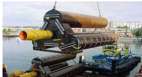
Fig 1 A Cluster of suction anchors adapted from [6]
