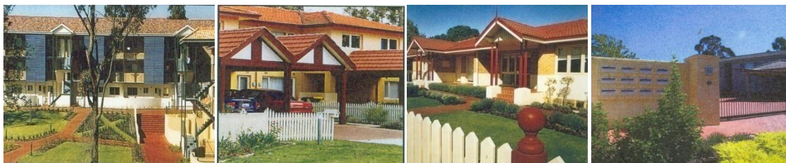
Images 20: Refurbishment of townhouses and individual properties
