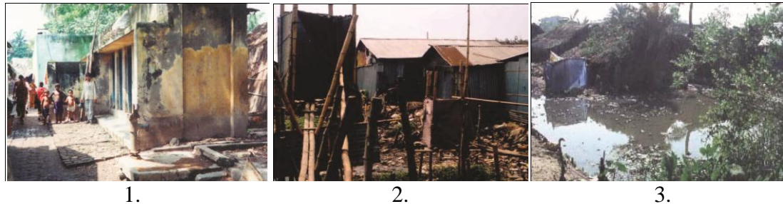
Images 15: Absence of sanitary facilities
