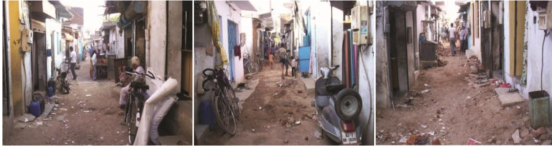
Images 7: The process of construction and repair of roads and pavers
