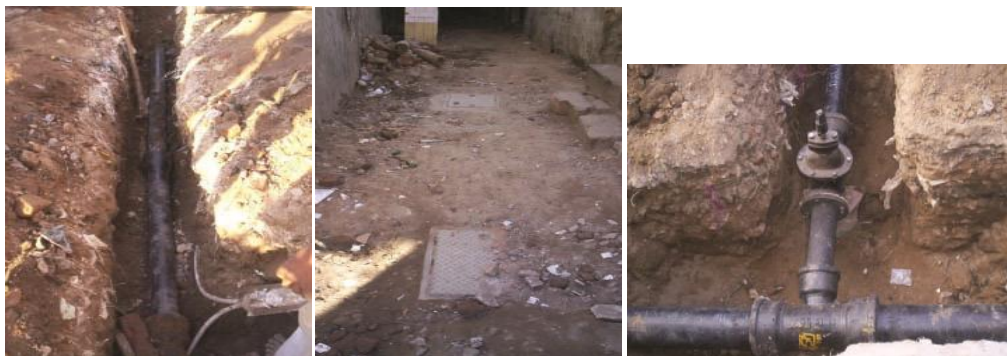
Images 8: Laying of pipes for water supply, solid waste chambers, and connection to underground waste water and storm water management
