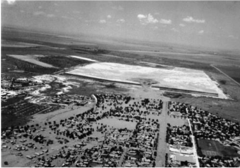
Figure 1.3 Aerial photograph of the Merriespruit tailings dam failure (Fourie, Blight, & Papageorgiou, 2001)
